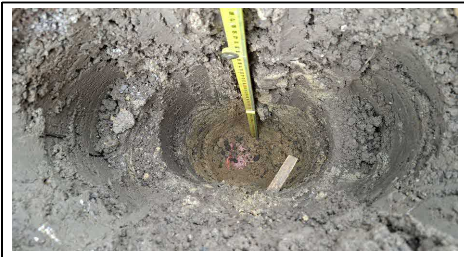
Plot 46 recording presence of membrane at base of clean cover system.
