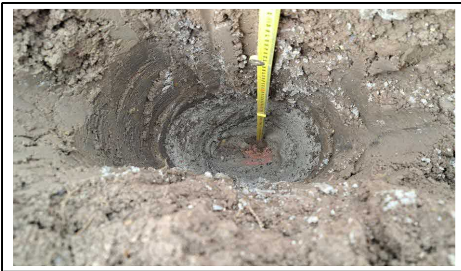
Plot 49 recording presence of membrane at base of clean cover system.
