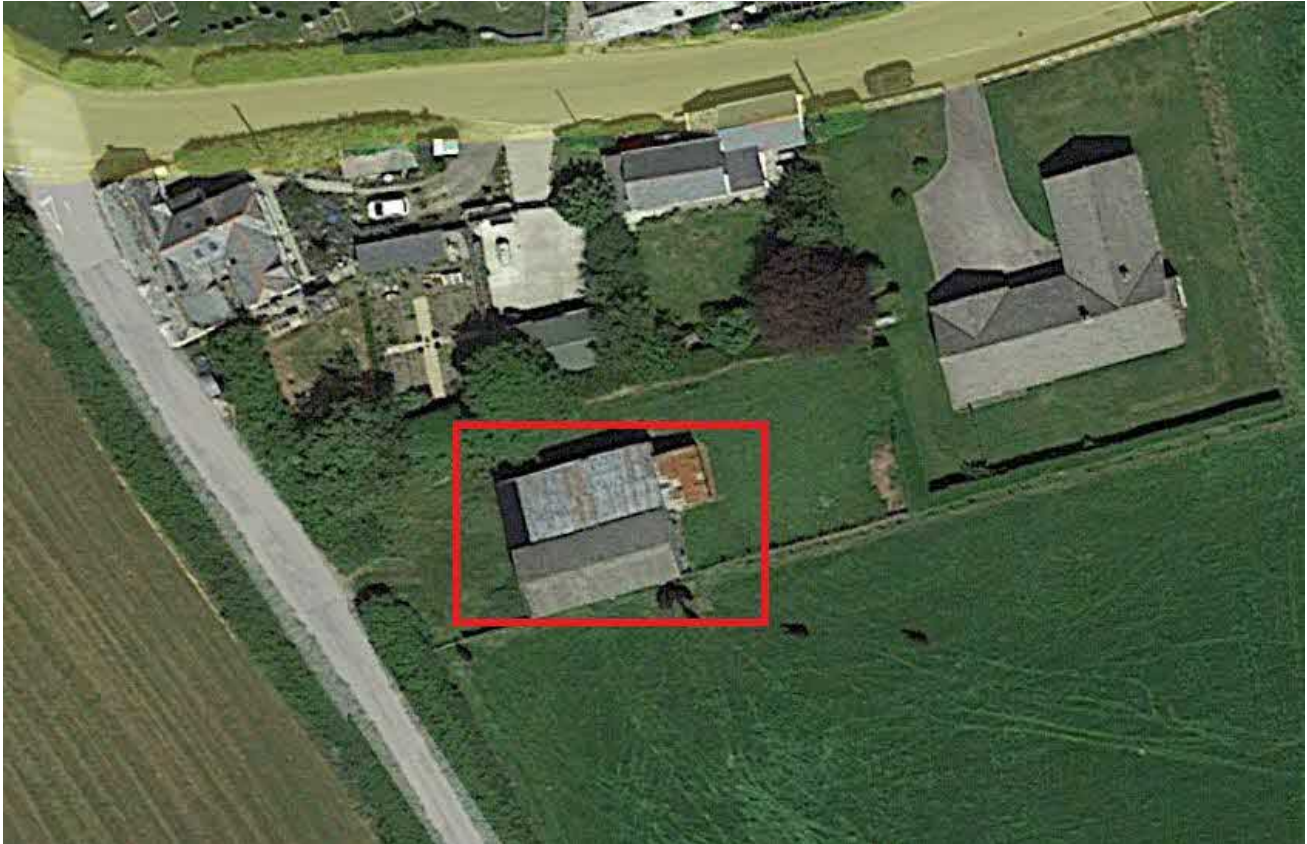
Above: Barn A (highlighted within red box)
