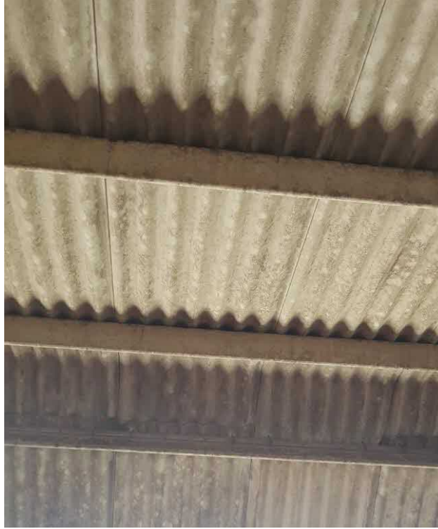
Above: Roof cladding to concrete framed section
