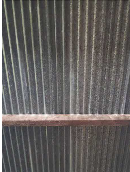
Above: Metal corrugated roof cladding, lean too roof
