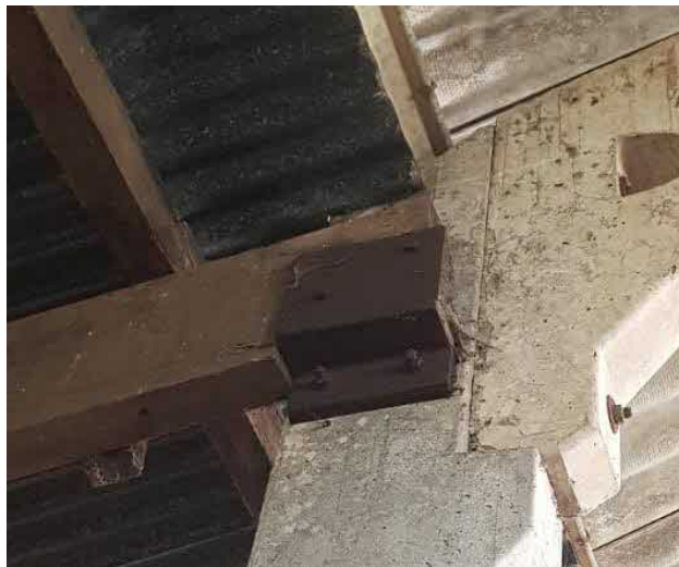
Above: Cleated connection support to principal timber rafter
