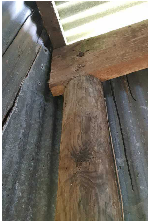
Above: Timber post with direct bearing over to principal timber rafter
