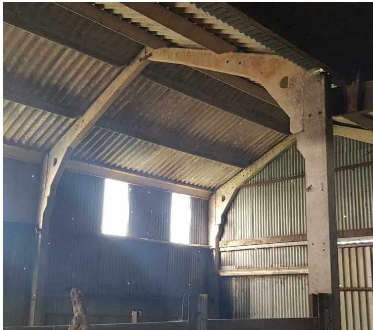
Above: Pre cast concrete portal frames
