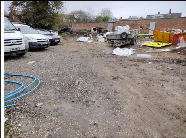
Photo 1: Area of unsealed surfaces used as parking
