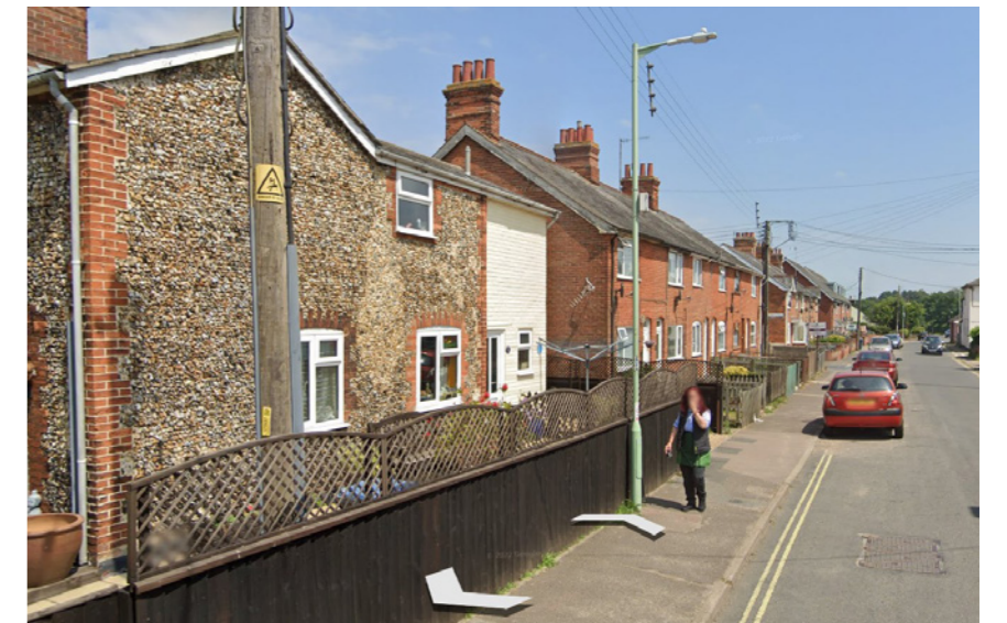
6) View along Valley Road- Residential buildings to the east of the site
