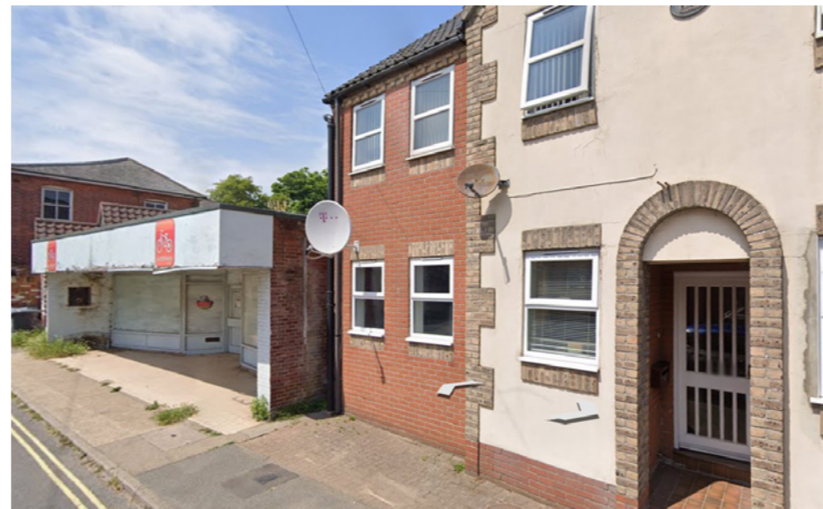
5) 5- 7 Valley Road front facade & 1 to 7 Valley Court in the foreground
