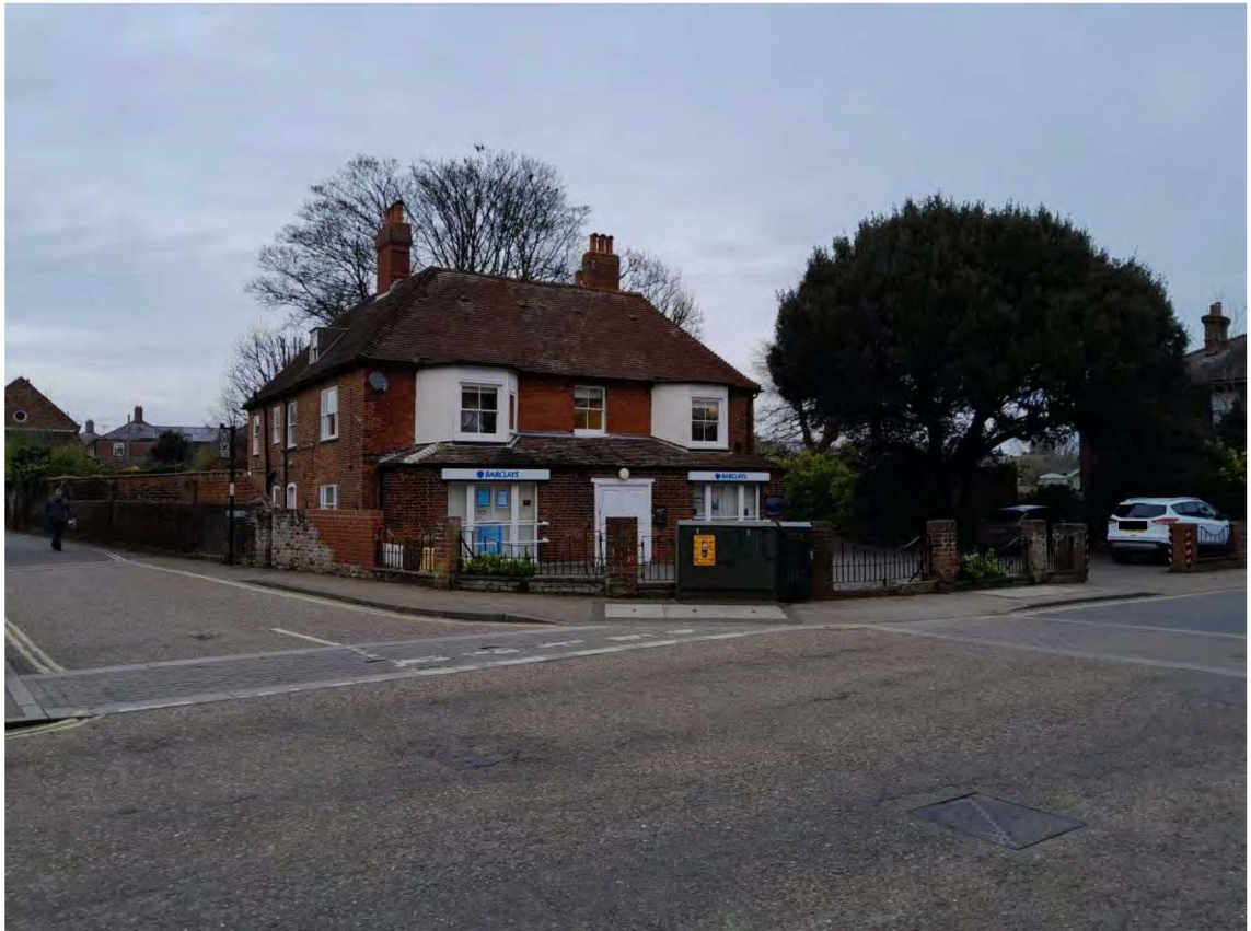
Plate 20: View of Barclays Bank from Main Street
