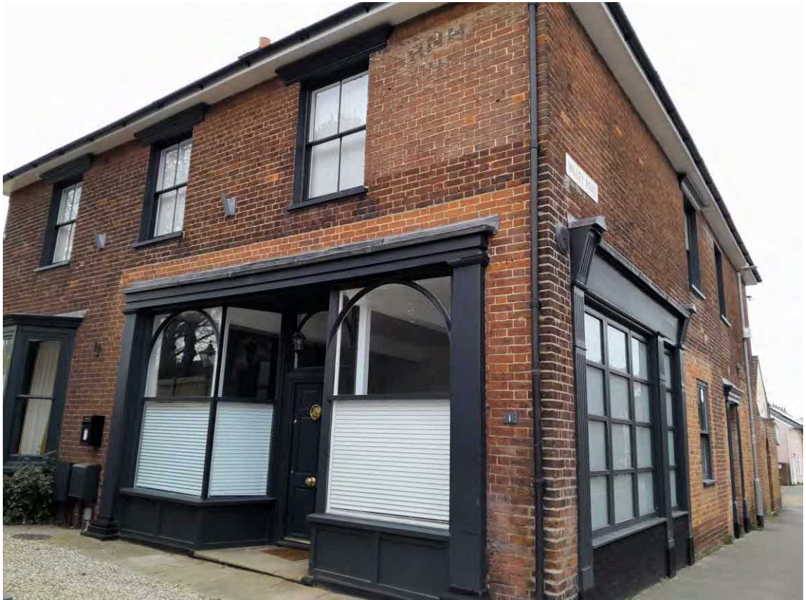
Plate 16: View of Veldor House, taken from Valley Road
