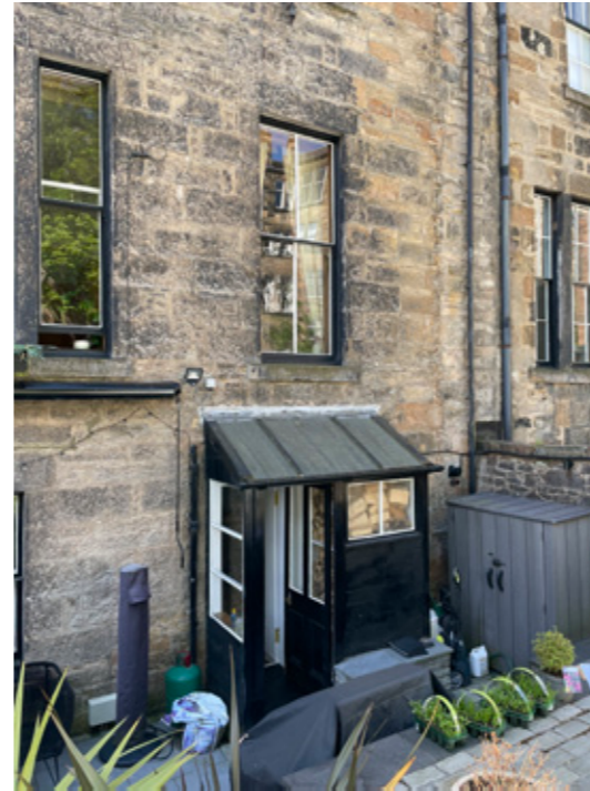
• existing access to rear garden
