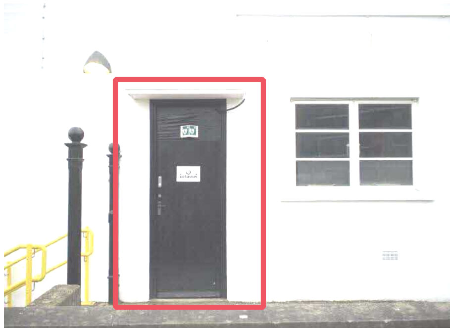
Fig. 16 Photo of existing opening on SE facade to be widened
