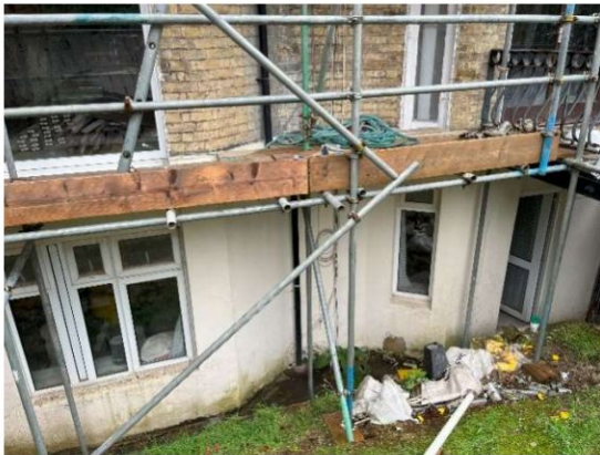
Out of character uPVC windows/doors
