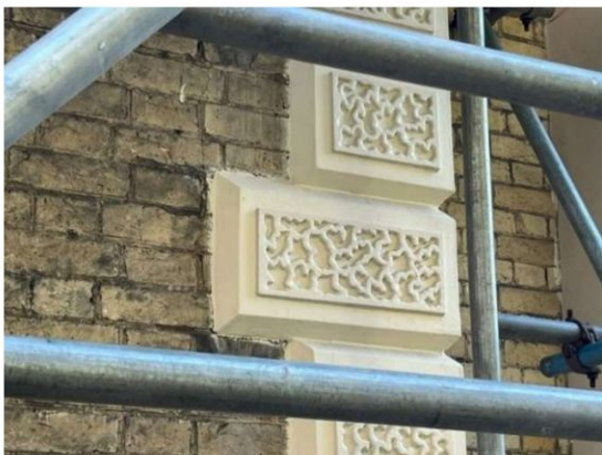
Detailed stone sets to corner returns.
