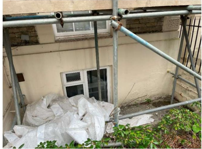
Lightwell directly outside kitchen
