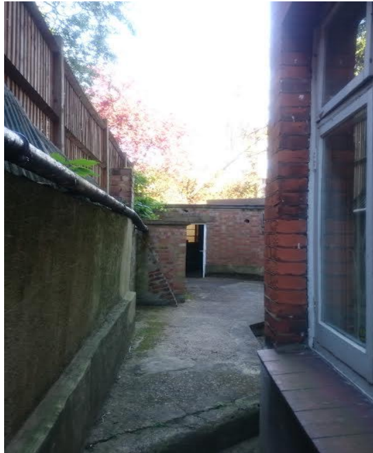
Image 3. Old Boiler Room Access and Exterior West Facade.
