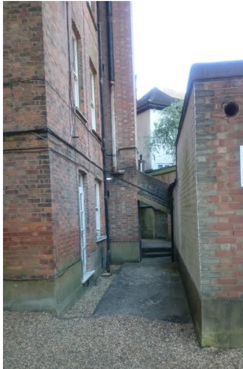
Image 5. South walkway showing relationship between Old Boiler House and existing Mansion Block windows.
