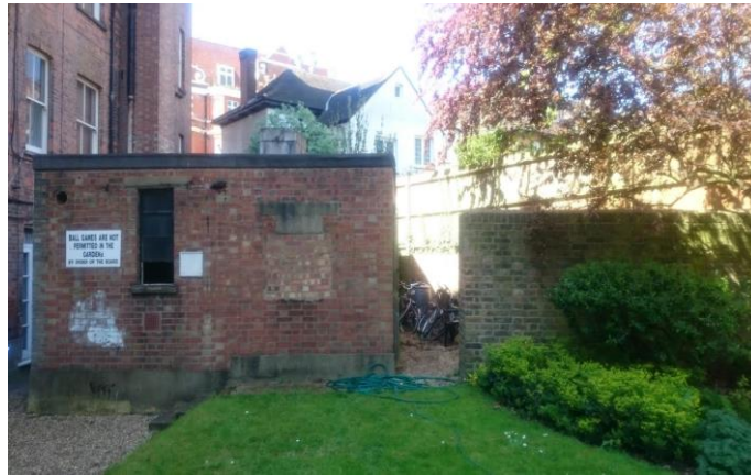
Image 2. Old Boiler Room Exterior East Façade.
