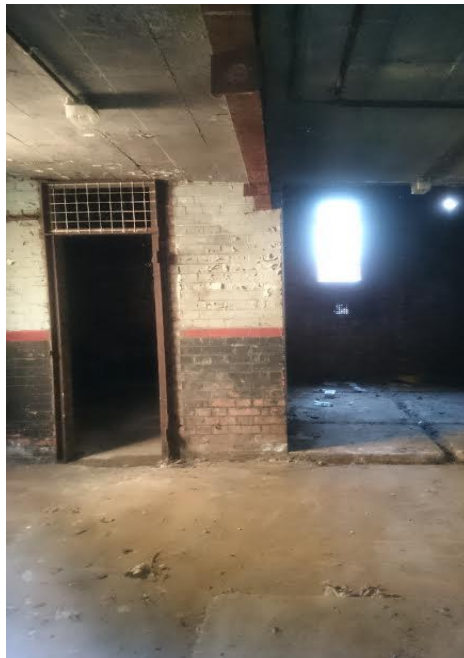
Image 1. Old Boiler Room Interior. View to tank platform.
