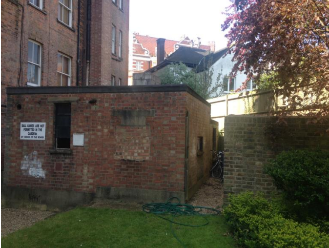
Figure 2: Existing front façade of the Old Boiler House
