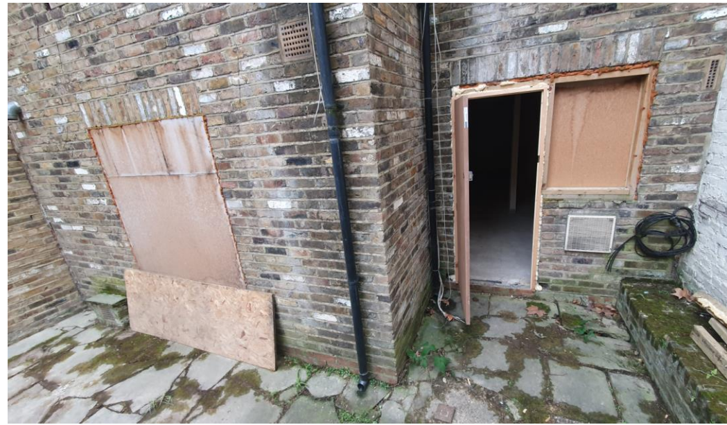
Door from Kitchen EL16 to Rear Lightwell EL20.
