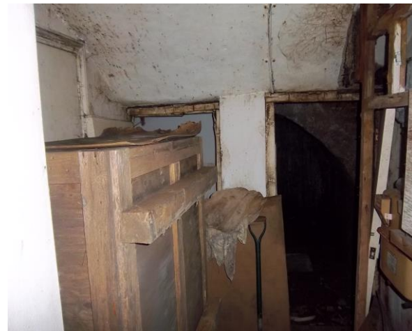
Vaulted ceiling in Lobby EL03 on Lower Ground Floor.
