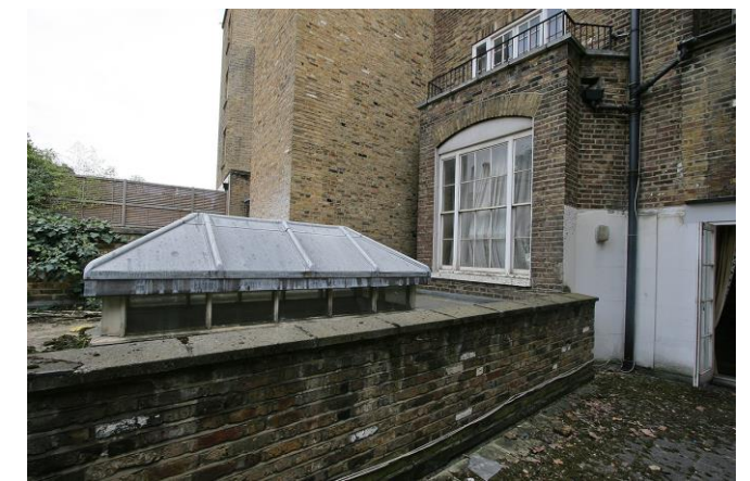
Flat roof and lantern over east part of rear extension
