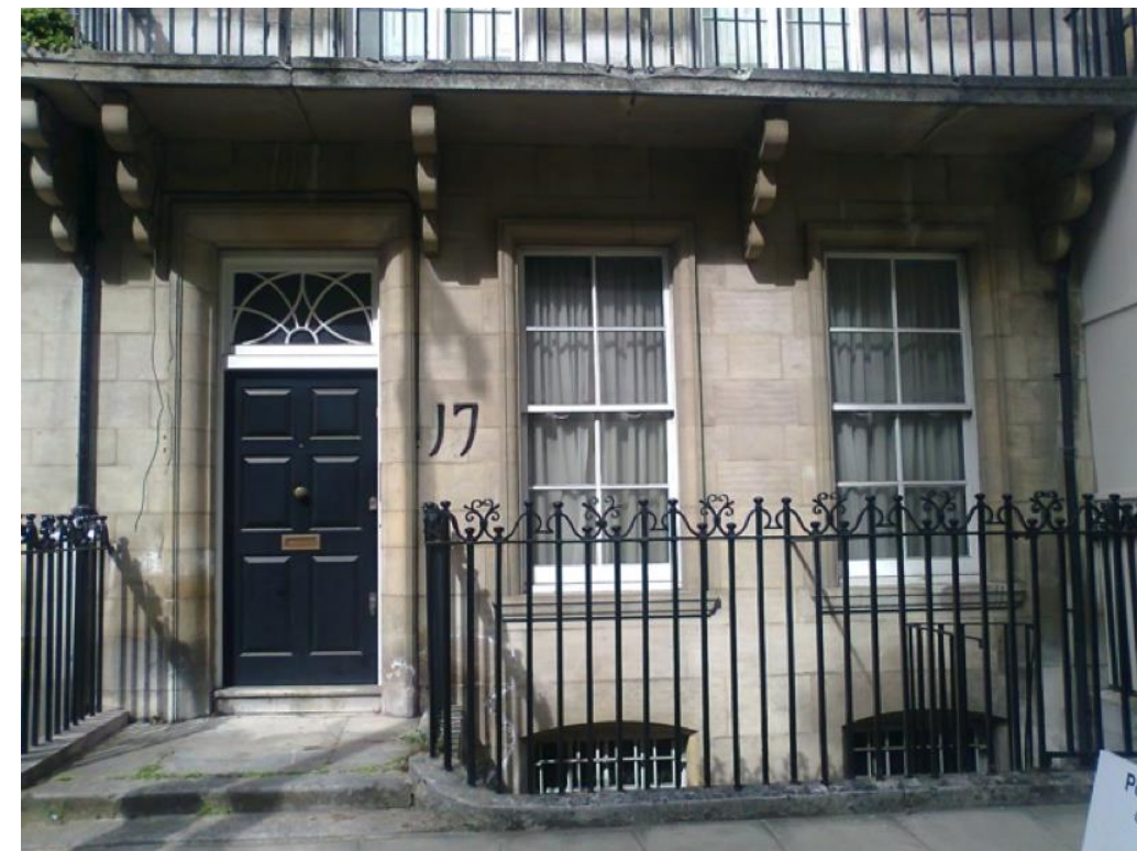
Main entrance door and gate to front lightwell.
