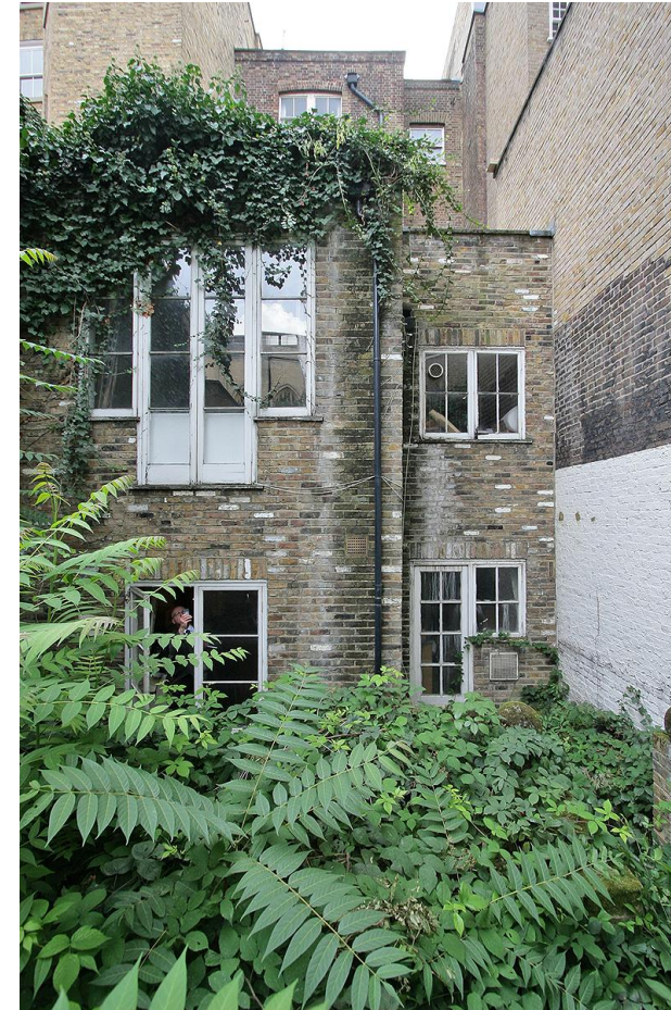
Existing rear extension.
