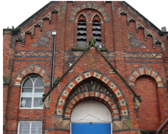
Brick at the rear of the Design Centre
