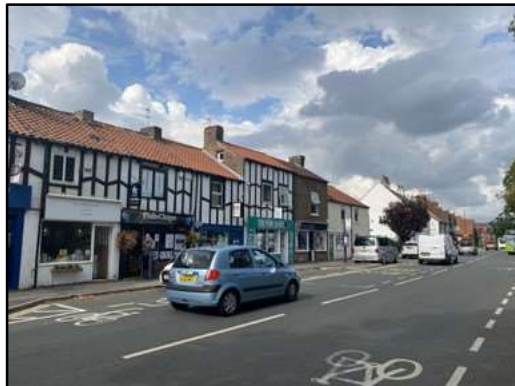
Front View of the Property from Street
