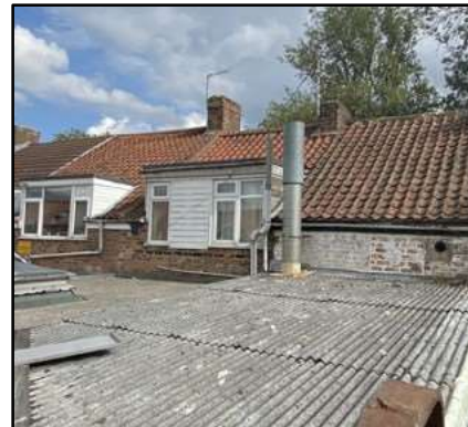
Rear of the Ground Floor Roof
