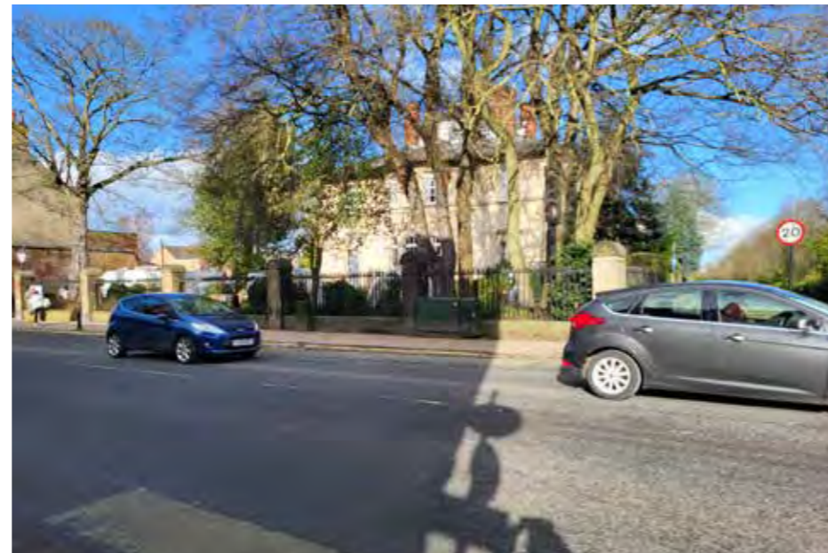
Figure 5.19 Photograph of the pods in situ, from Bootham Road. There are seven temporary pods and the revised proposals seek permission for five pods, of the same design as those in situ, for a temporary period.
