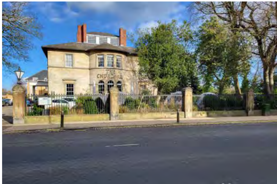
Figure 5.17 Photograph of the pods in situ, from Bootham Road. There are seven temporary pods and the revised proposals seek permission for five pods, of the same design as those in situ, for a temporary period.
