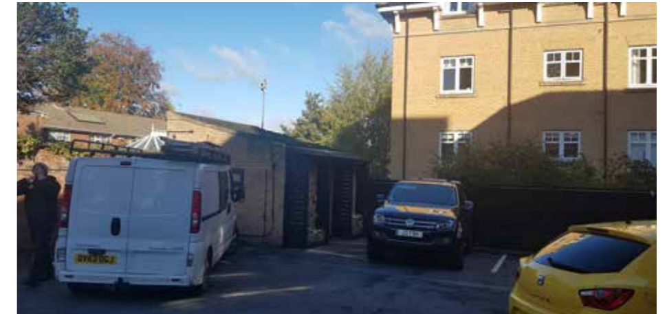
Figure 4.5 The rear of the Churchill Hotel, showing the detracting Grosvenor House
