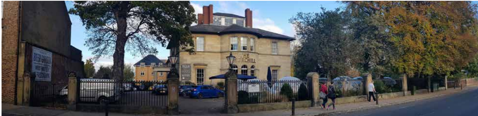
Figure 4.3 Stitched photograph of the listed building showing its setting to the south, as seen from Bootham (source: The Landscape Partnership)
