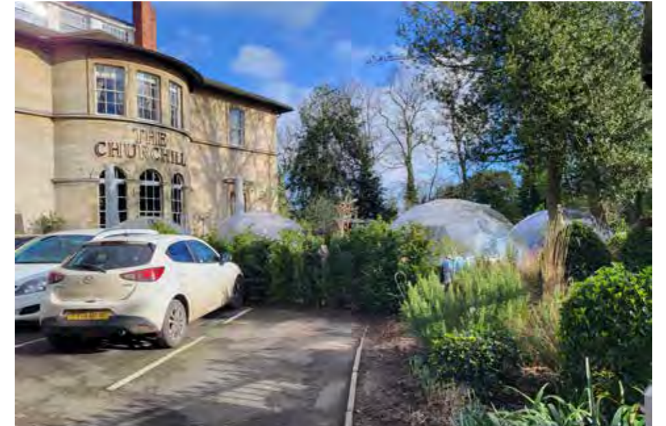
Figure 5.20 Photograph of the pods in situ, from the hotel entrance gate on Bootham Road. There are seven temporary pods and the revised proposals seek permission for five pods, of the same design as those in situ, for a temporary period.
