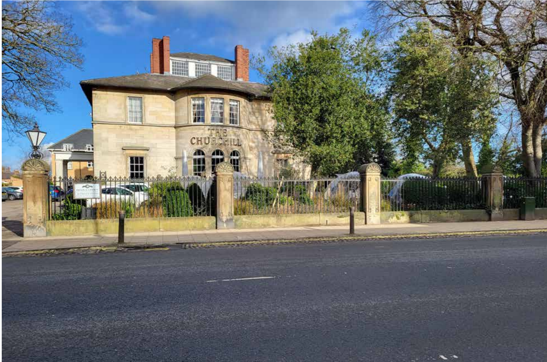
Figure 1.2 Recent Photograph of the Churchill Hotel. 7 temporary pods are visible in the front garden.
