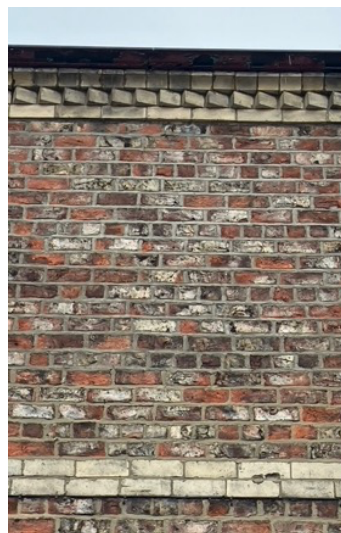
Plinth for raised ground level White brick string course and eaves detail
