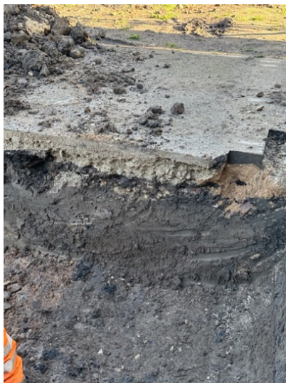
Site Photograph March 2024 – clean horticultural soil
