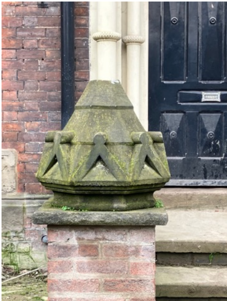
Existing stone feature on brick pier at 126 Fulford Road
