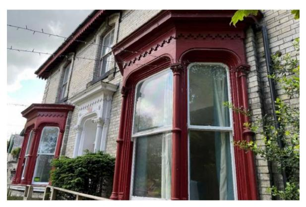
The proposal would involve the repair and redecoration of the existing window frames in the front elevation of the building including the existing sashes being replaced with new timber sashes in a matching painted timber design with heritage double glazing.
