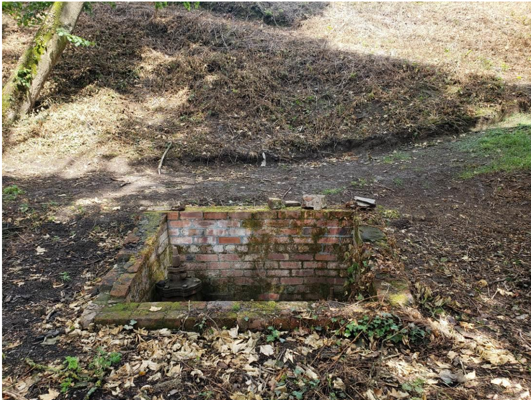
Photograph 9 – Redundant infrastructure confirming brownfield use
