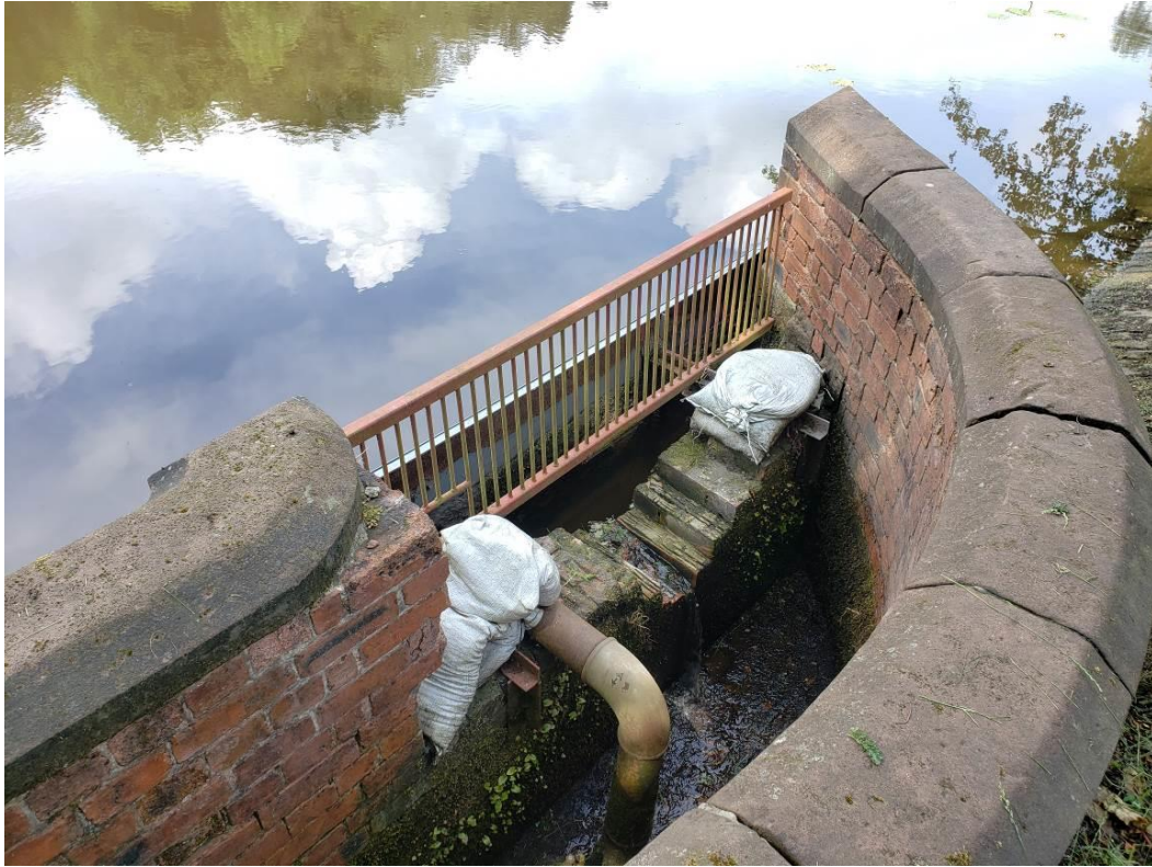
Photograph 8– Existing dam overflow weir
