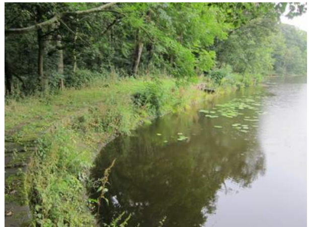
6 – Right abutment return embankment
