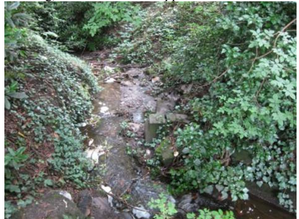
27 – Water course downstream of headwall
