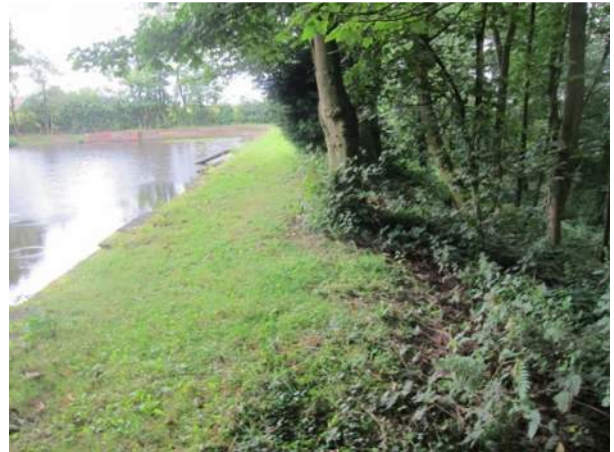
2 – Downstream embankment crest from right
