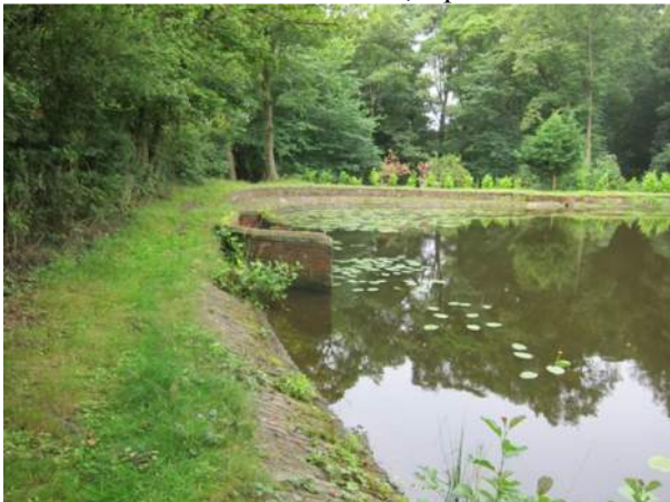
15 – Overflow B to left and A to right
