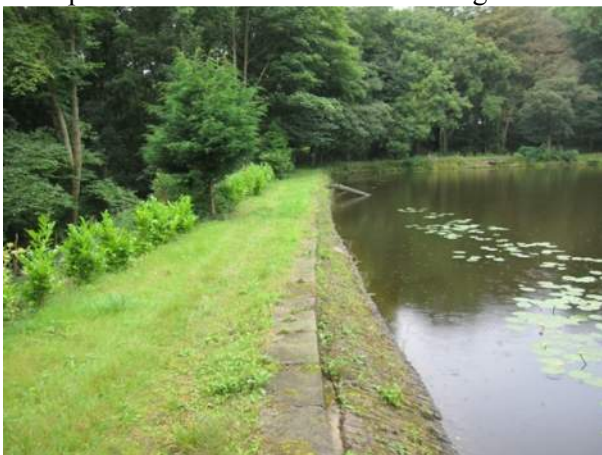
3 – Upstream embankment crest from left
