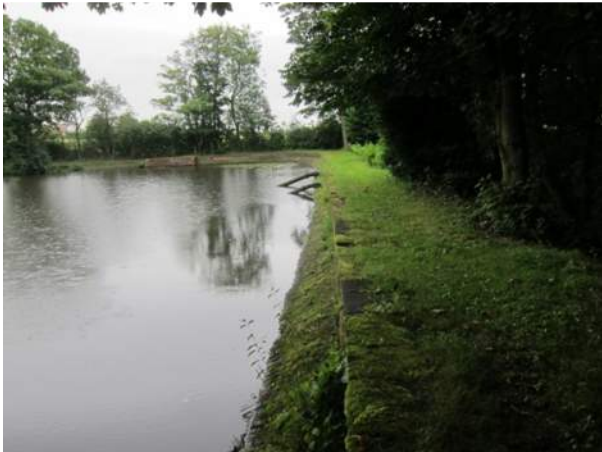
1 – Upstream embankment crest from right
