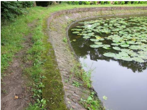
5 – Left abutment return embankment
