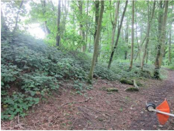
7 – Downstream embankment face from right
