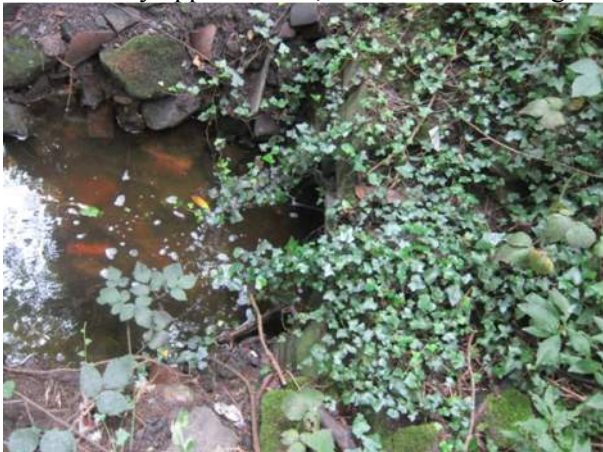
26 – Discharge headwall downstream of road
