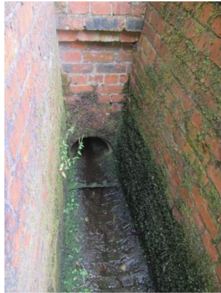
16 – Overflow B – chamber outlet
