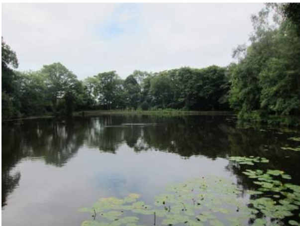
11 – Embankment upstream face
