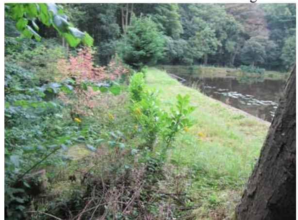
4 – Downstream embankment crest from left
