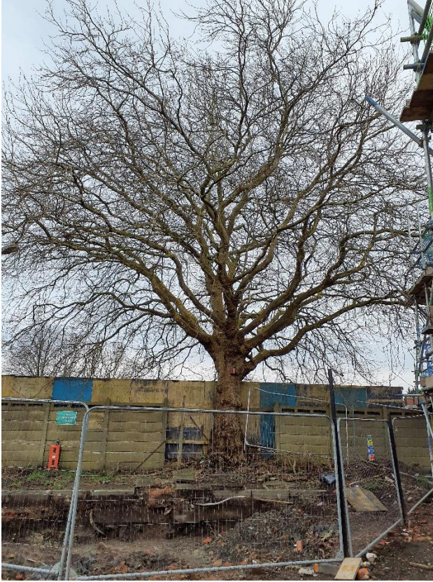
Figure 5 T23 with tree protection fencing installed, after tank removal.
