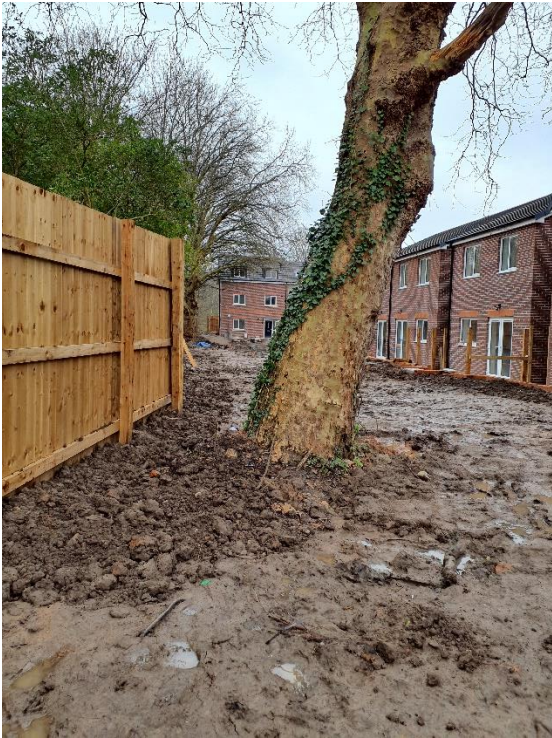
Figure 3 T9 Backfilled with a heavy clay-based soil.
