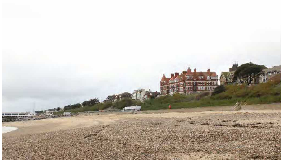
Plate 9. View towards Colchester Institute Main Building from the beach
