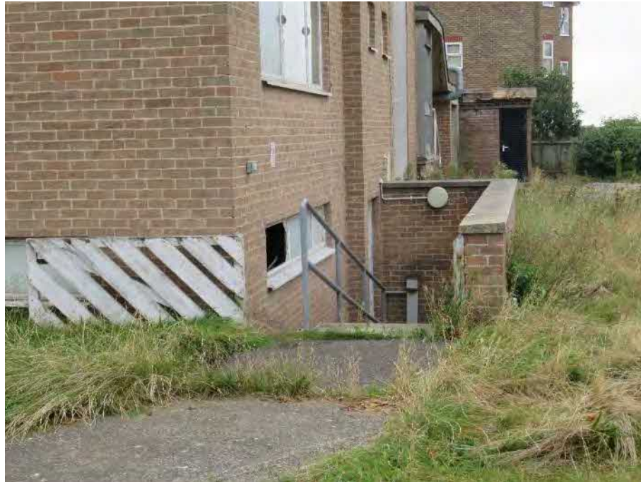
Plate 3. View of basement level
