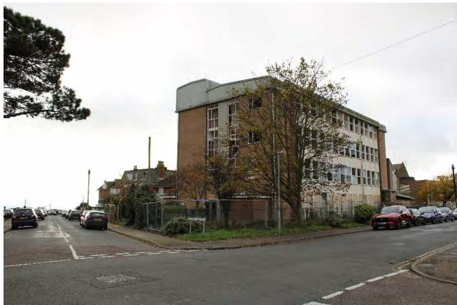
Plate 1. View towards the Site from the north east
