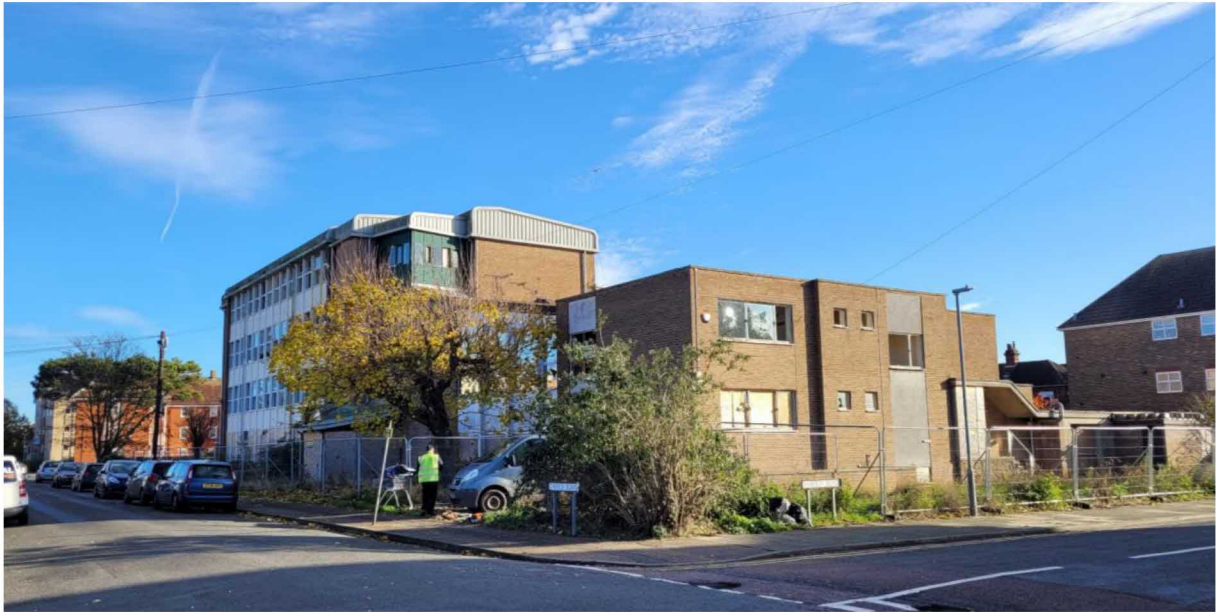
North western side of the Site.
