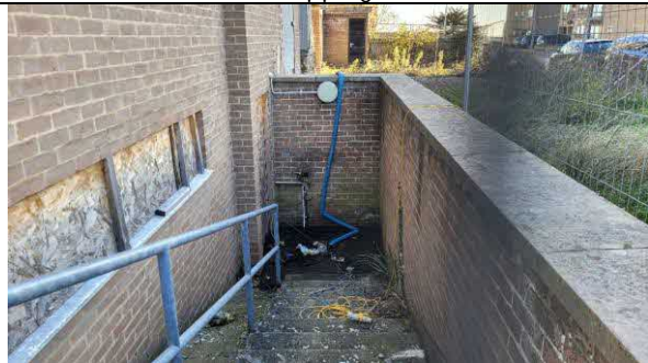
Photo 29: Slope on the western side of Building 1.
