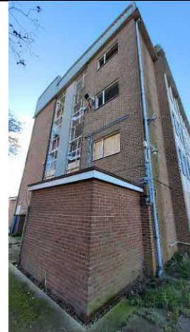
Photo 10: One storey section on the eastern aspect of the Building 1.
