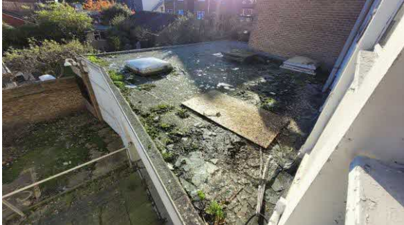
Photo 27: Felt roof on one-storey section on the southern side of Building 1.
