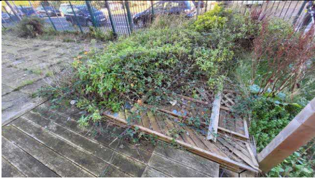
Photo 9: Decking, wooden fencing debris and a pond beneath
