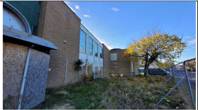
Photo 2 Northern aspect of the building.
