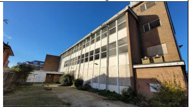
Photo 12: Southern aspect of Building 1 with car park.
