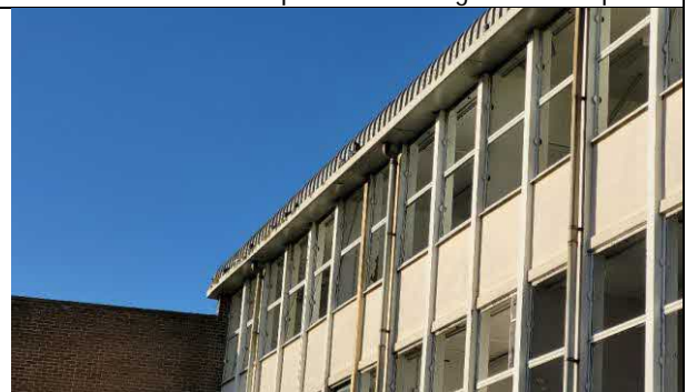
Photo 14: Feral pigeons perched along the soffit box on the southern aspect.
