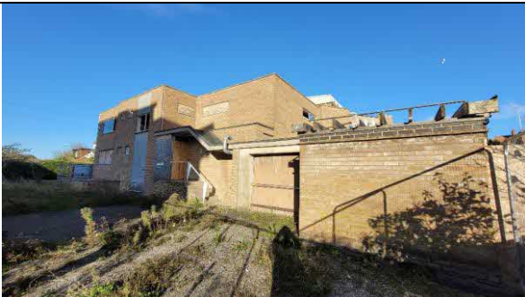
Photo 28: Western aspect of the Building 1, with a garage extension.
