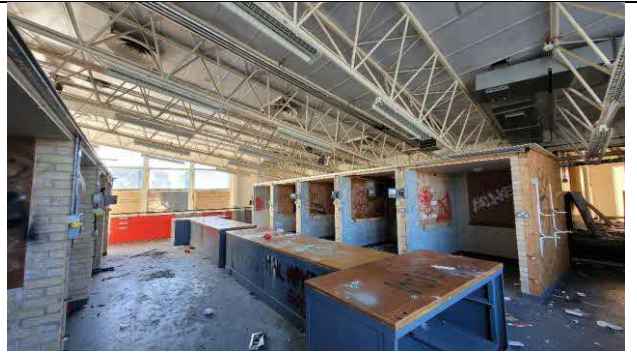
Photo 24: Fourth floor with exposed rafters and ceiling.
