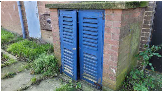
Photo 11: Electrical box on the eastern aspect of Building 1.
