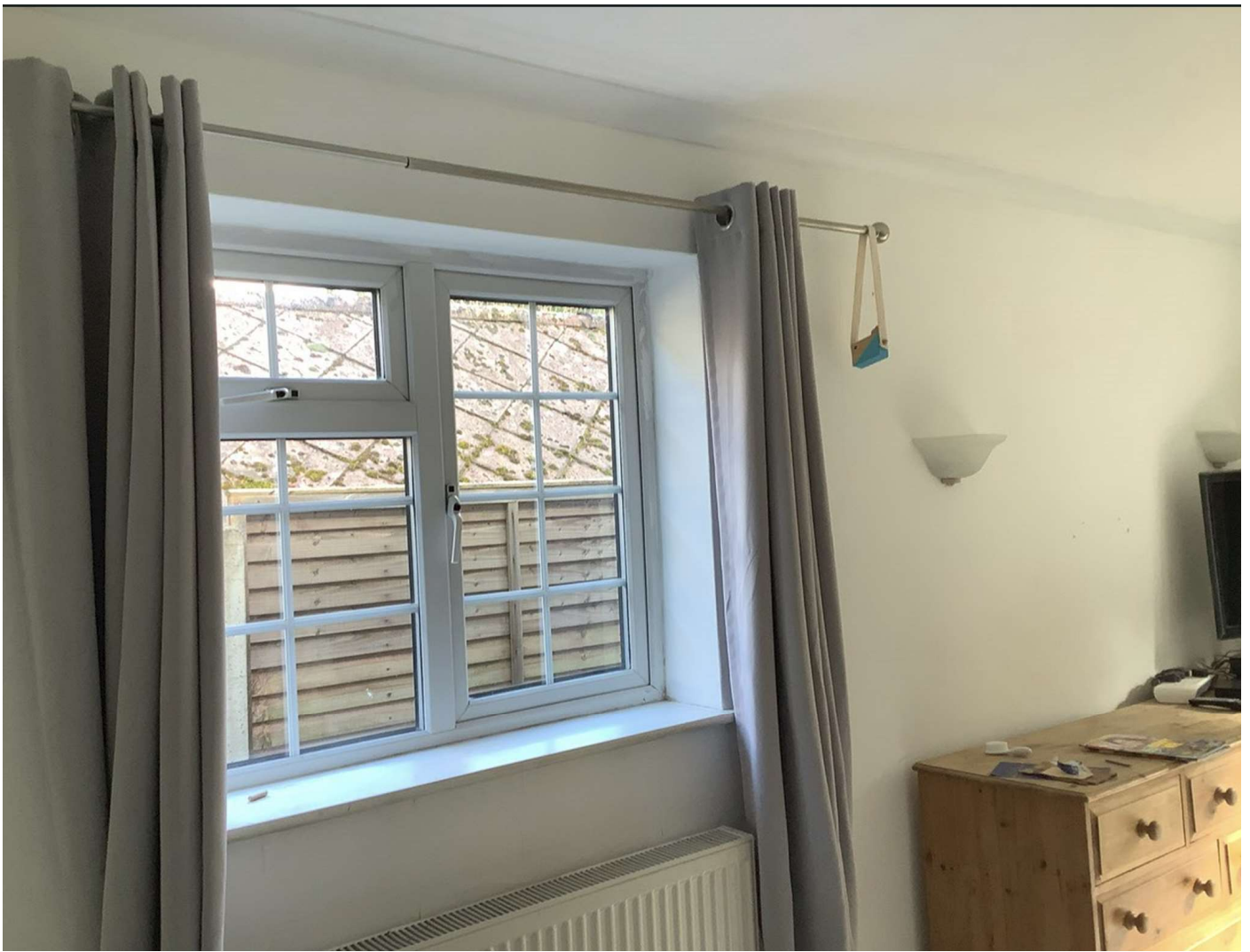
Figure 4a: Existing Side Window to Bedroom 2 – New Side window to garage to match this one.
