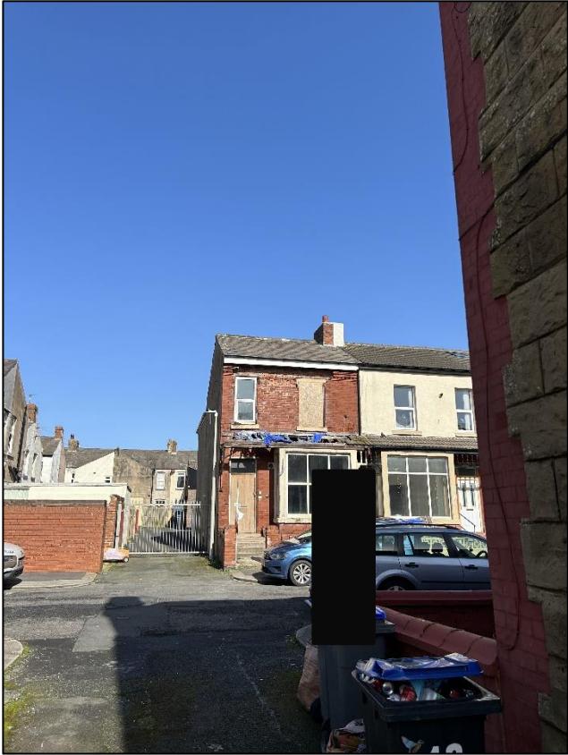
Plate 1 – The southern elevation of the structure on site
