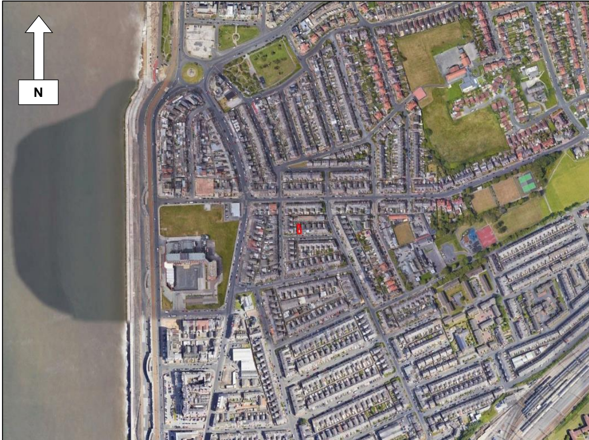
Figure 5.1 – Location of the red line boundary within the landscape © Google Earth Pro 2023/24
