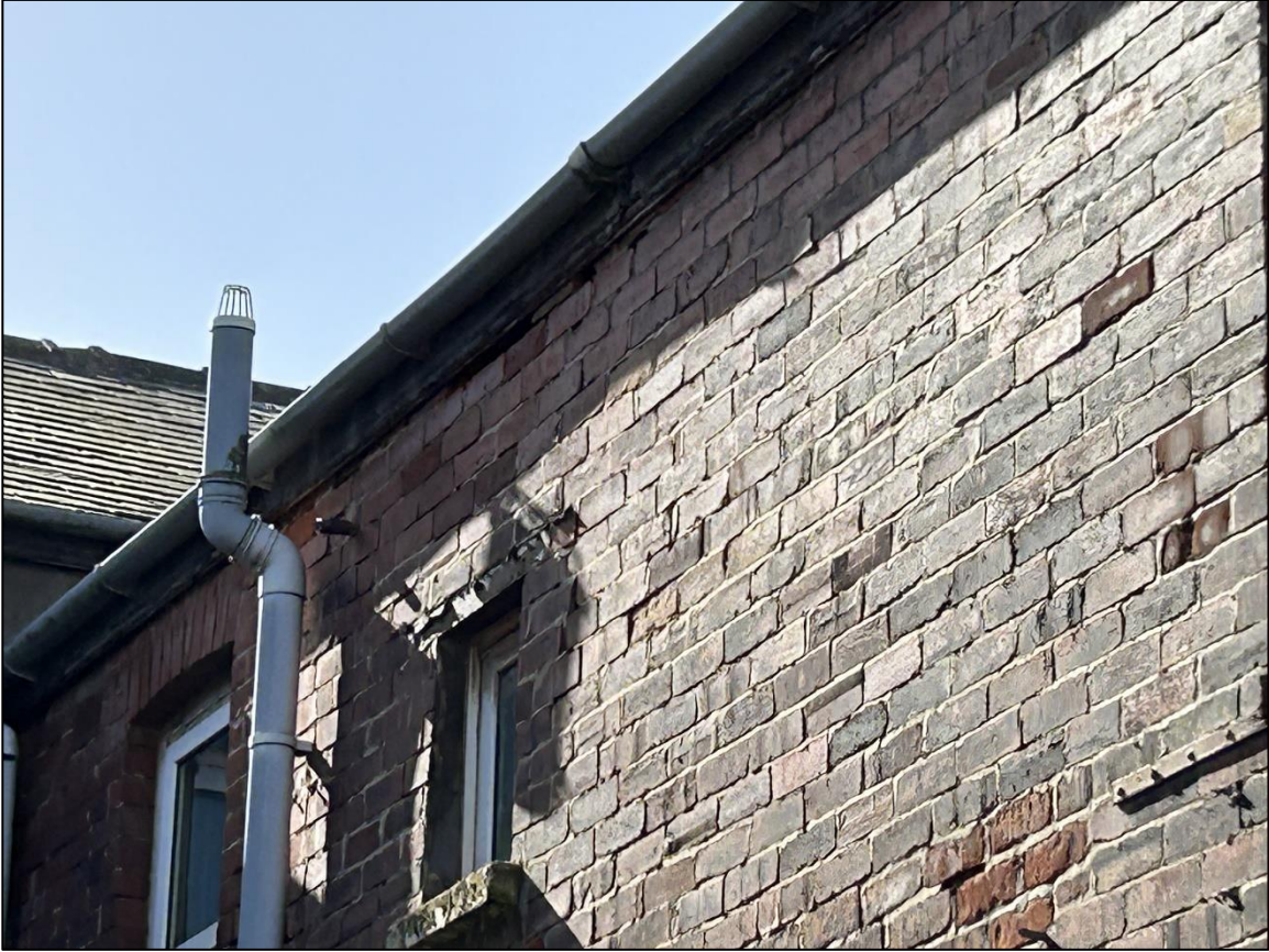
Plate 7 – Close up of lifted fascia
