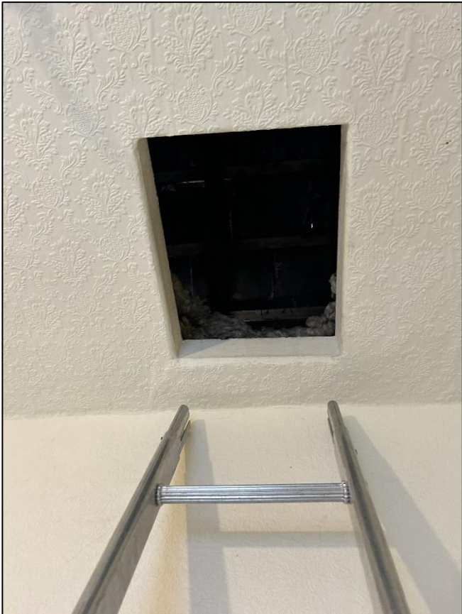
Plate 10 – Access hatch for L1
