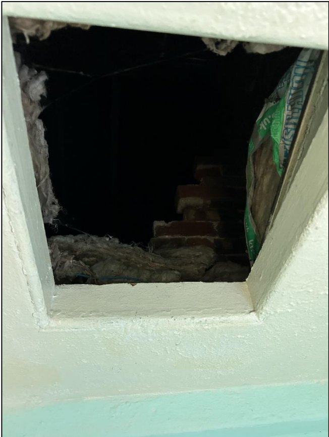
Plate 12 – Access hatch for L2
