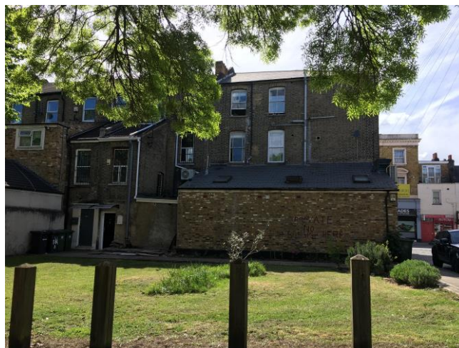
Rear of 182-186a Deptford High Street looking west at junction with Albury Street and Mary Ann Buildings towards Deptford High Street
