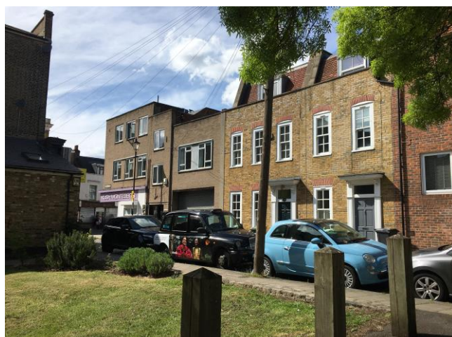
190-196 Deptford High Street and 1-5 Albury Street looking north-west at junction with Albury Street and Mary Ann Buildings towards Deptford High Street
