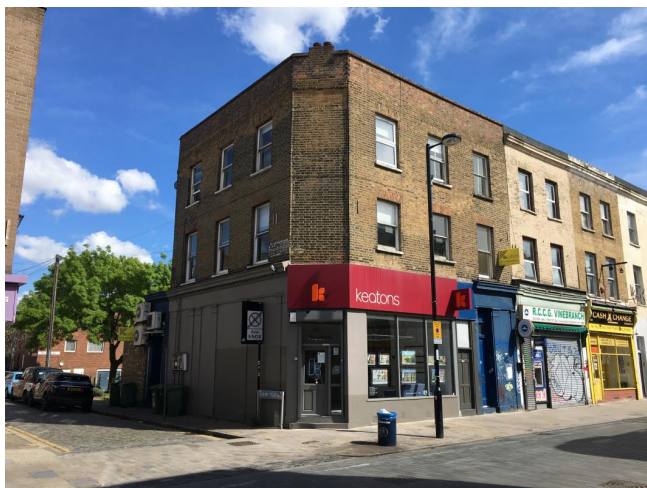
182-186a Deptford High Street looking south-east at junction with Albury Street
