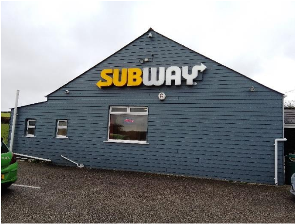
Photograph 3 – View of the east aspect.
