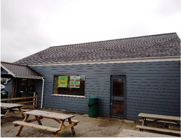
Photograph 1 – View of the north aspect of the building.
