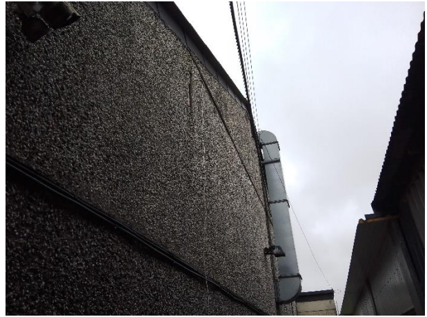
Photograph 4 – View of the west aspect.
