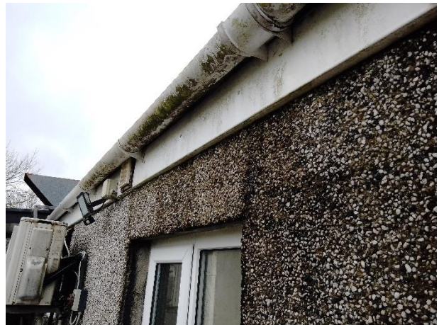
Photograph 4 – View of the mostly well sealed bargeboards.
