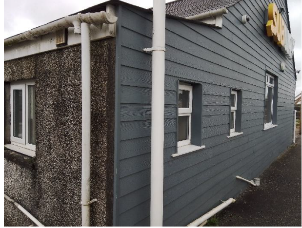
Photograph 2 – Closer view of the extension to be removed.
