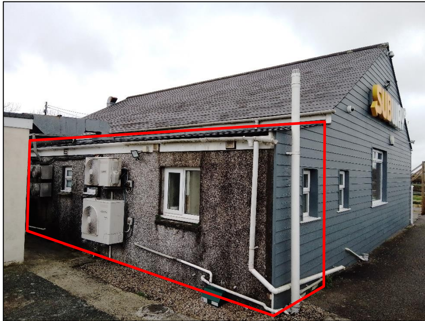
Photograph 1– View of the south aspect where the extension is located.
