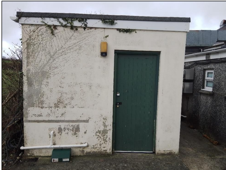
Photograph 1– View of the east aspect of the utility outbuilding.
