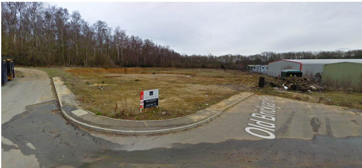
Fig 2. View across site taken from northeast corner of the site, looking down the previously constructed access road.
