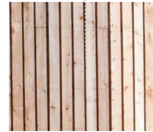
Scotlarch vertical rainscreen cladding
