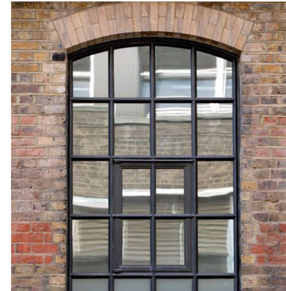
Image 69: Example of metal windows to north river wall
