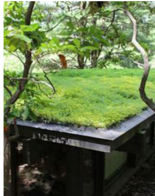
Image 71: Example of green roof to boat house
