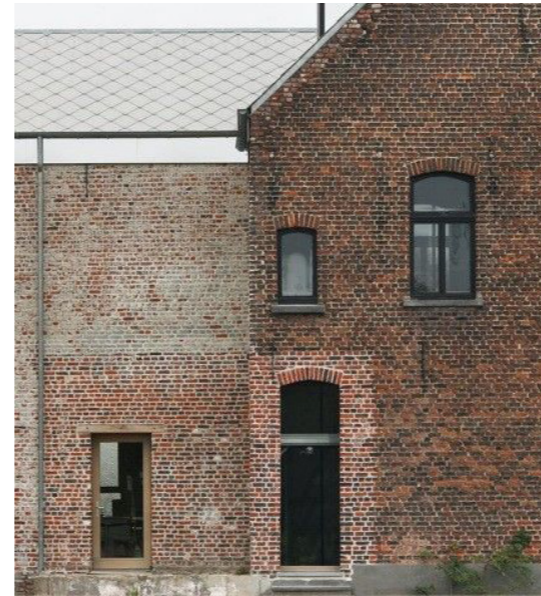
Image 68: Example of masonry facades re adaptation north river wall servants cottage
