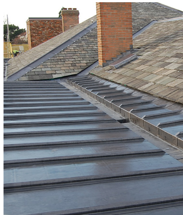
Image 70: Example of lead and slates roof coverings to outbuildings
