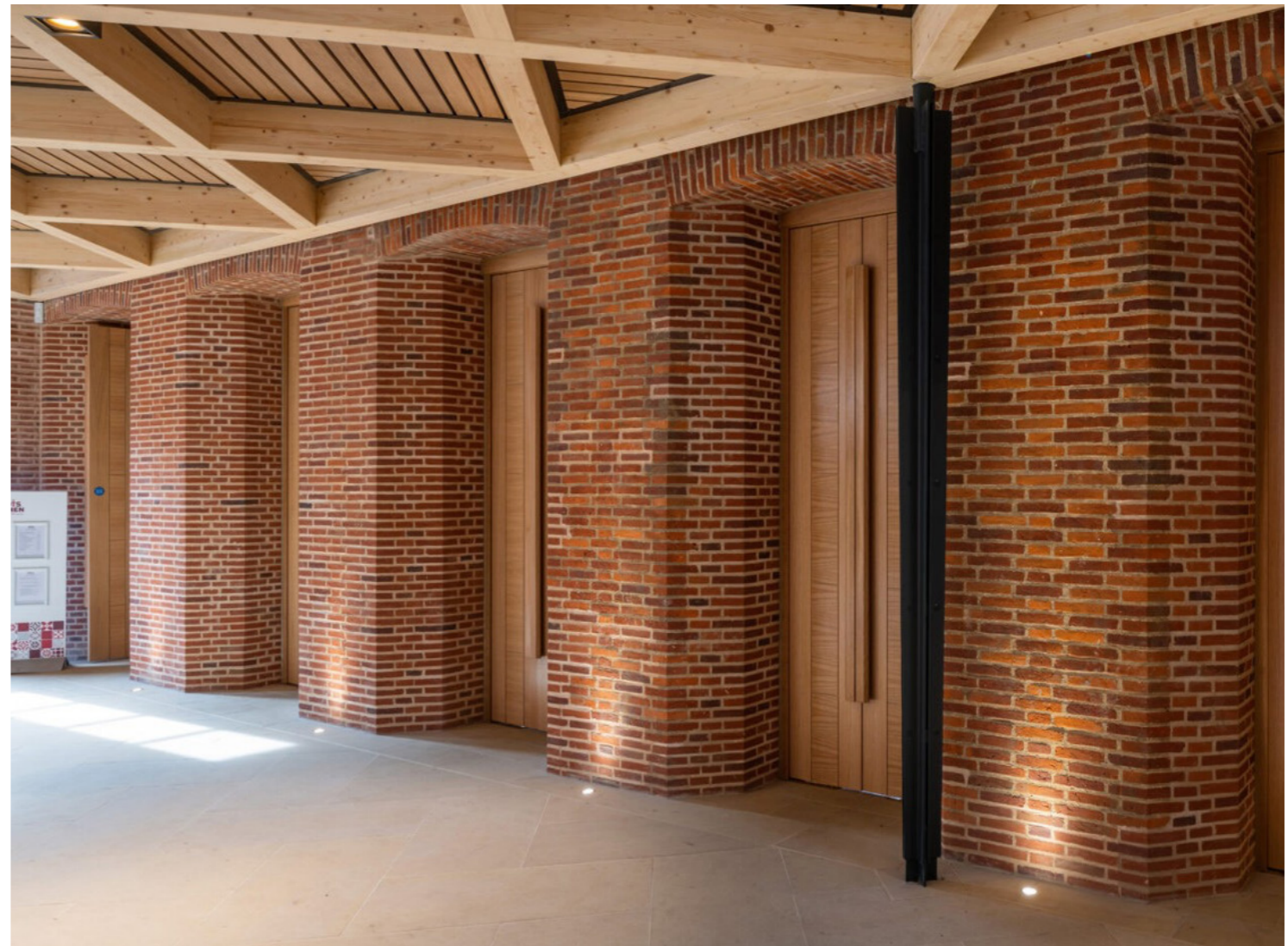
Image 63: Example of exposed masonry walls, stone floors, timber fixtures and exposed timber structure to ceilings in circulation areas and larger common rooms.
