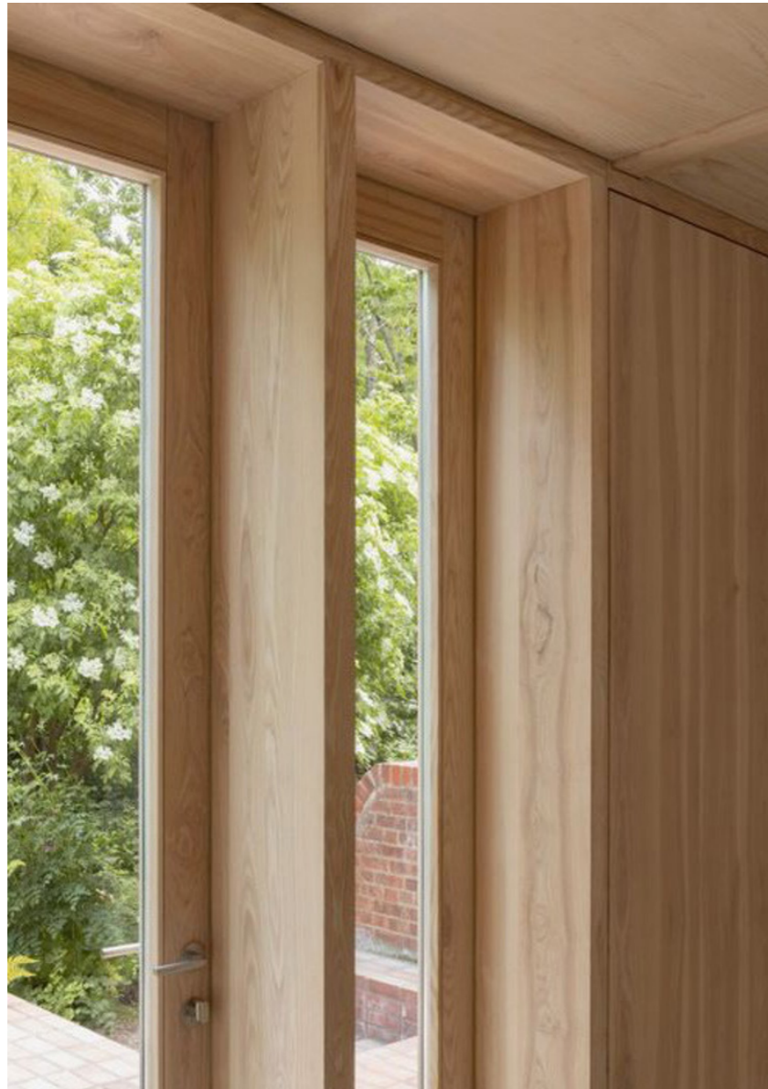
Image 64: Internal timber windows detail
