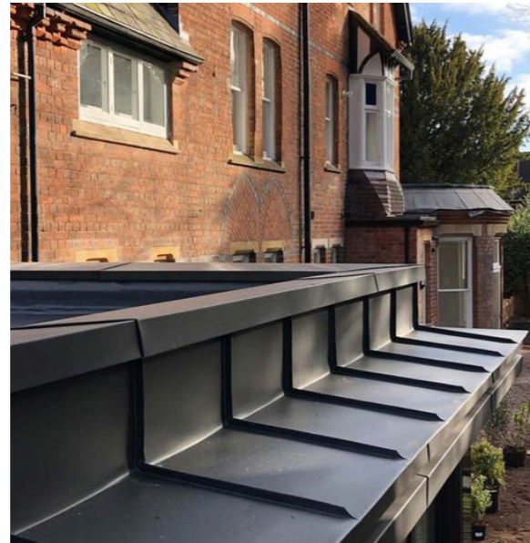
Image 67: Example of dark zinc roofing to entrance building
