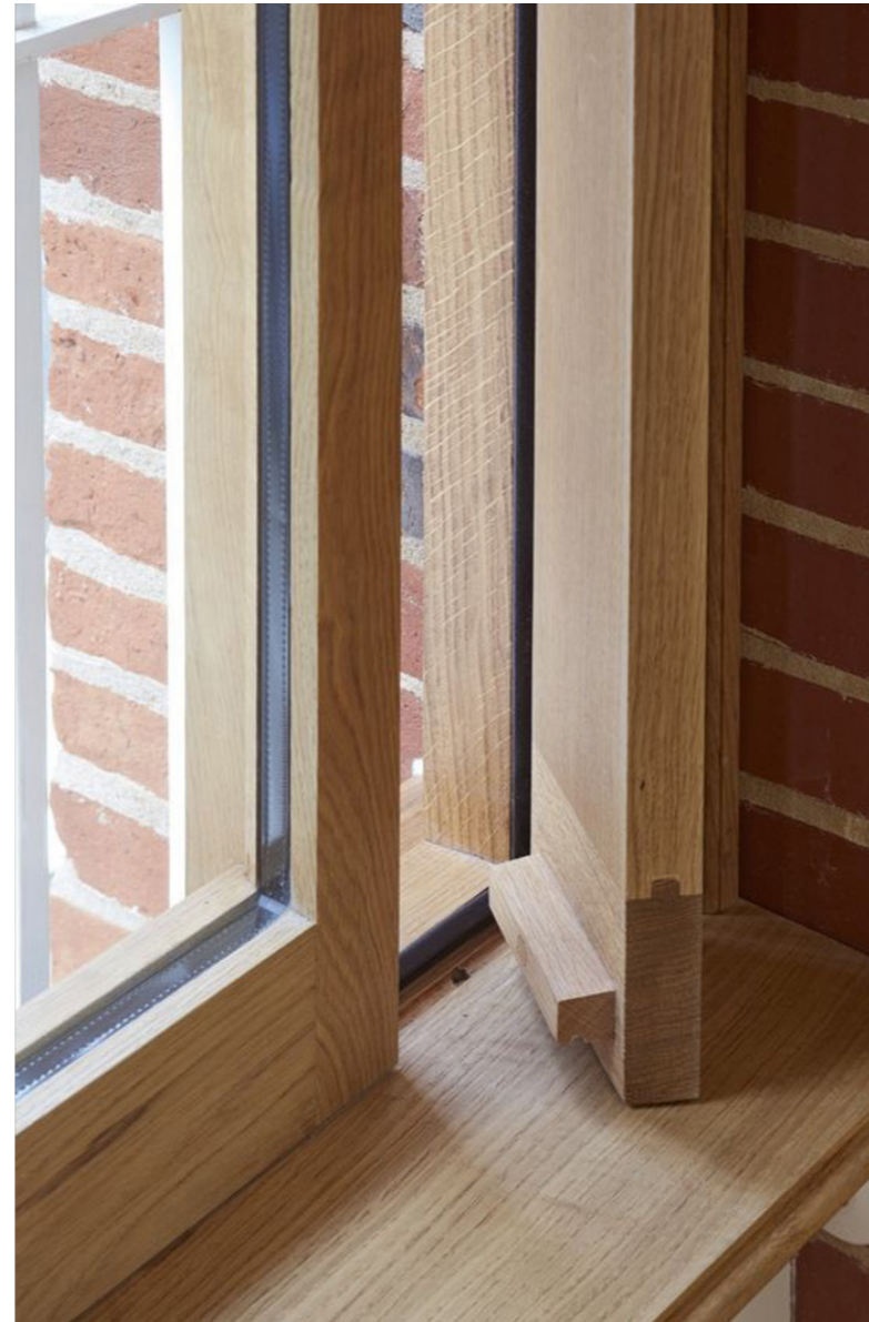
Image 65: Detail of timber windows
