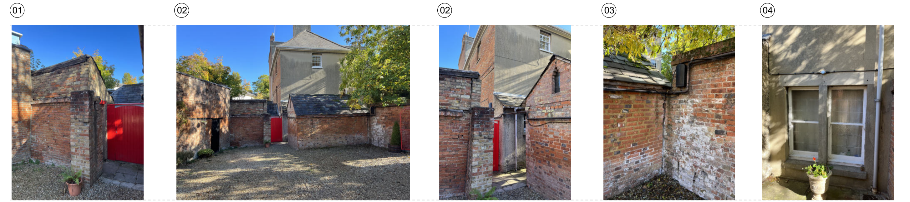
01 20th c. alteration to the historic service yard boundary wall extension and pier addition 02 View of the rear wing, Servants' cottage and historic outbuildings seen from the carriage yard 03 Detail view of historic outbuildings adjacent to the west facade of the rear wing 04 Detail view of the historic cycle store outbuilding at junction with the existing pedestrian pathway wall 04 Detail view of 20th c. later addition window opening
