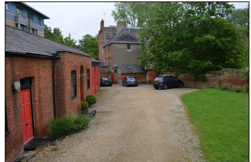
9) The existing driveway area will be re-surfaced with load bearing gravel (pea shingle). Cycle storage for resident will be provided adjacent to the existing brick wall on the south side of the driveway.
