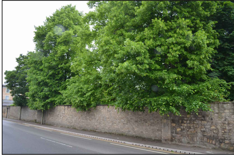
1) Specialist tree consultant Barrells have been commissioned to advise on appropriate protection of the existing mature trees.
