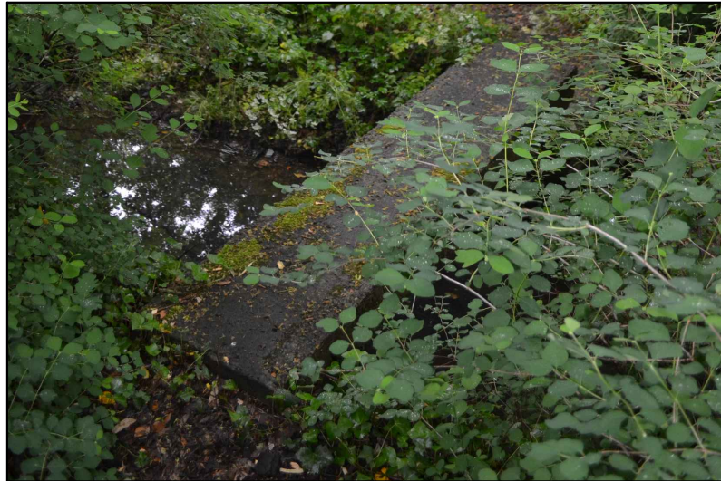
5) New links across the shallow streams will open up access to the Eastern perimeter of the grounds and complete new walking routes through the grounds.
