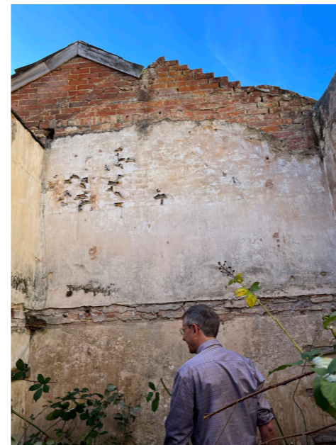
Image 35: View of ruined servants' cottage interior
