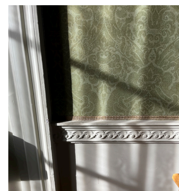
Image 29: East wing first floor south principal room dado detail
