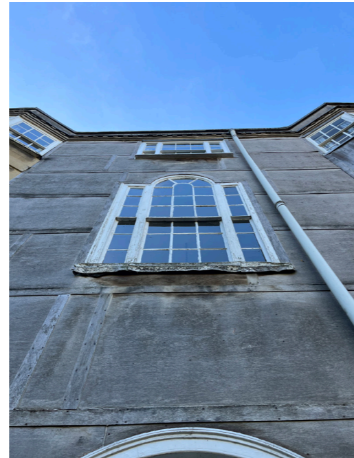
Image 31: West wing east elevation plywood paneling
