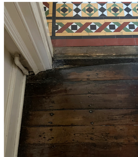
Image 28: East wing ground floor north principal room timber floor detail
