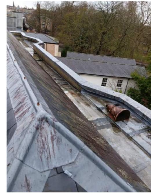
Image 33: West wing main roof showing slates and lead coverings
