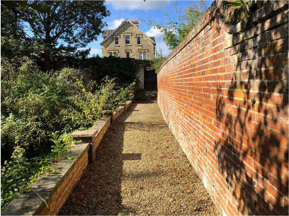
Plate 7: General view west along the walkway
