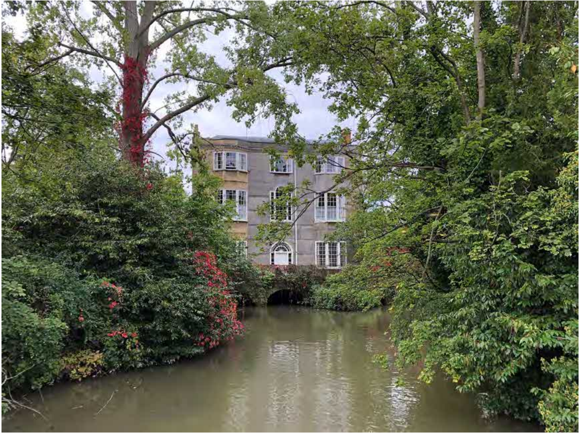
Plate 1: View looking west towards Grandpont House
