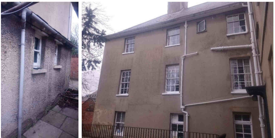
B5, 'extension' west elevation (north, L) and south elevation (west, R)
