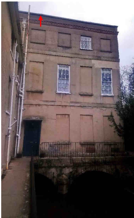
B5, west elevation (south) with gap under lead flashing and upper part of south elevation (east)
