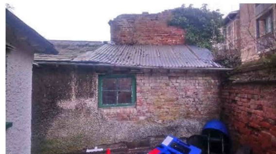
B4, west elevation incl. gap between wall and roof (L) and east elevation (R)
