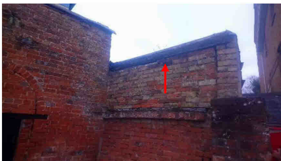
B4, west elevation incl. gap between wall and roof (L) and east elevation (R)
