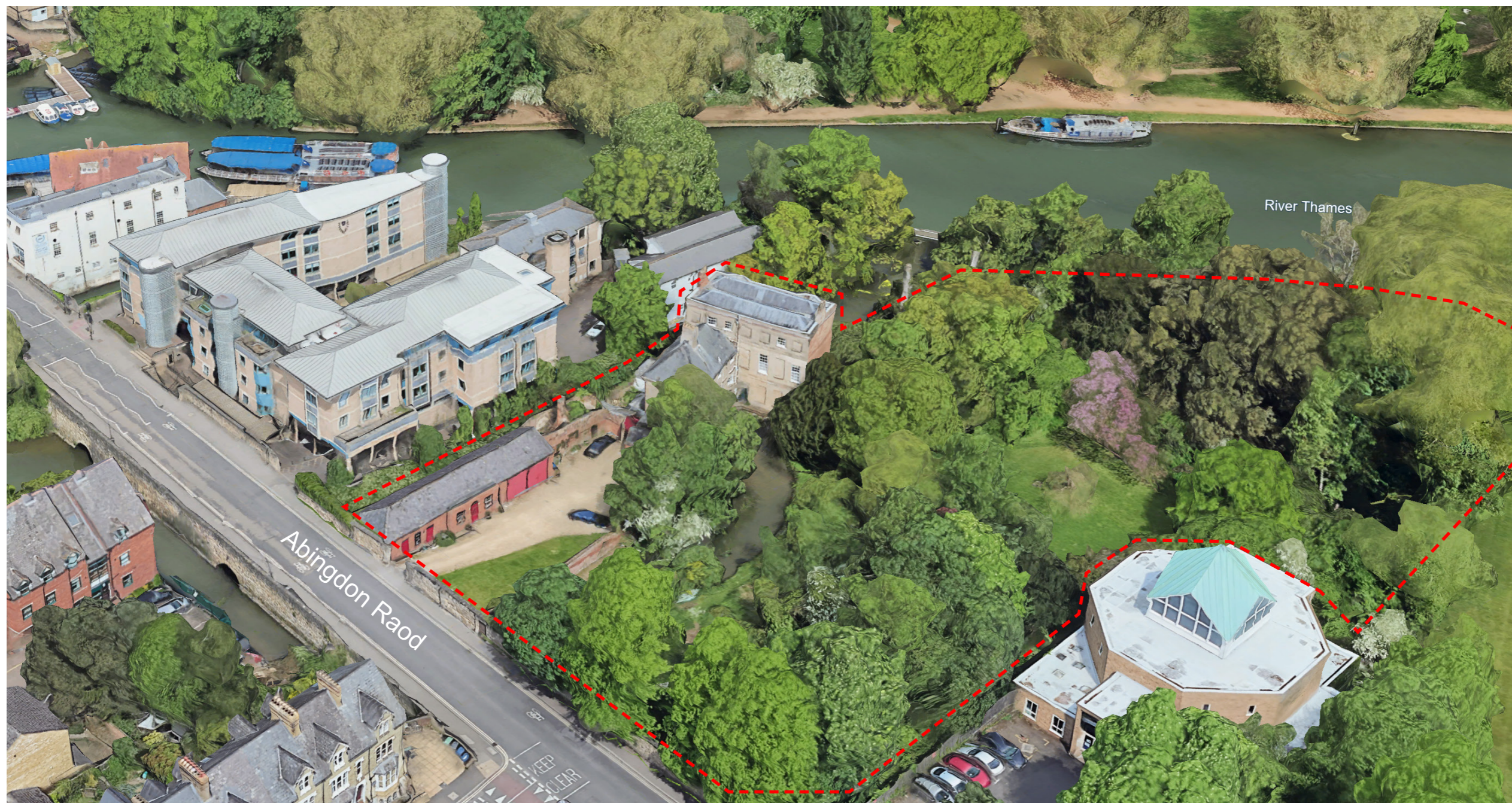
Image 2: Aerial view of Grandpont House
