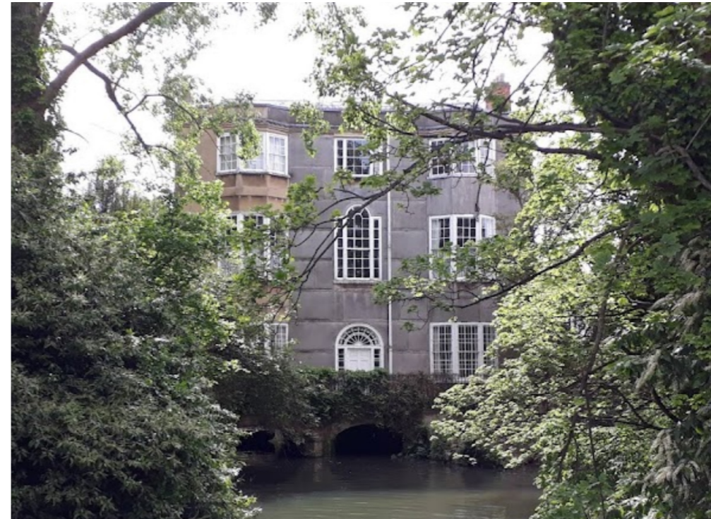
Image 7: East facade of the principal building
