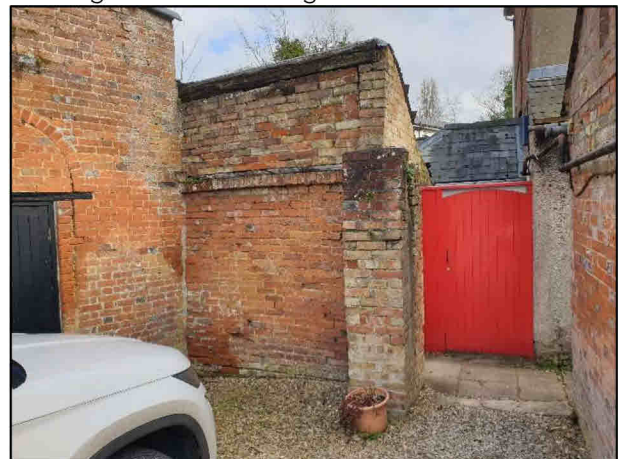
Building B4 – view looking north-east
