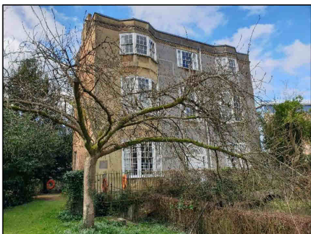
Building B5 (Grandpont House) – view looking north-west
