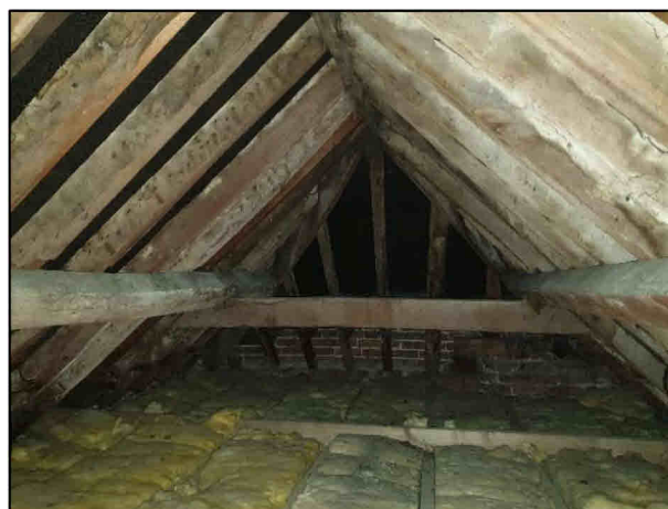
Building B5 (Grandpont House) roof void – view looking north
