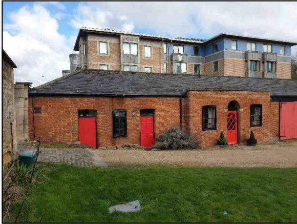
Building B1 – view looking north
