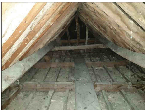
Building B5 (Grandpont House) roof void – view looking south
