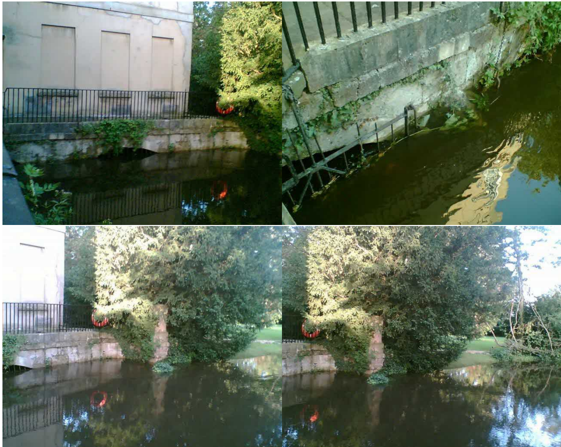
Figure 10: Photos of the flooding at Grandpont House in 2007.
