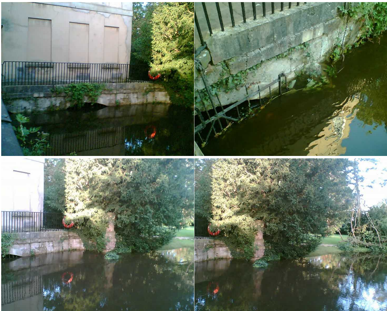
Figure 2: Photos of the flooding at Grandpont House in 2007.
