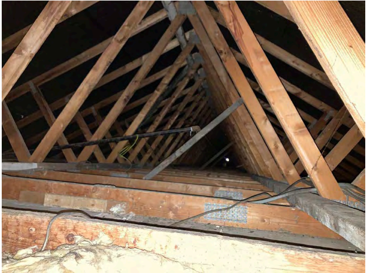
3.47 The modern roof of the outbuildings
