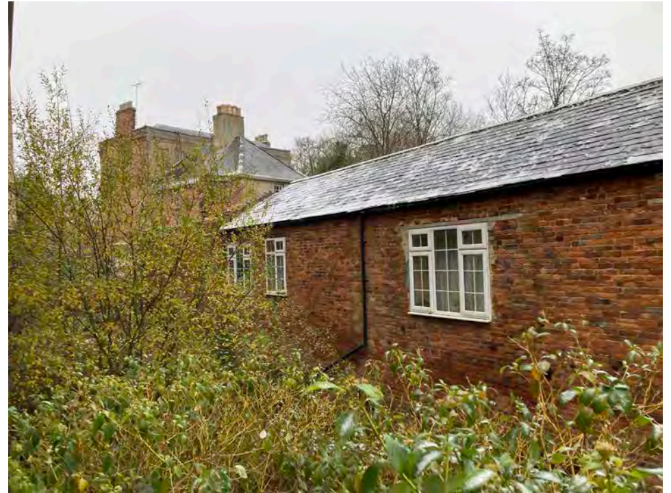
3.18 Part of the north wall of the outbuildings
