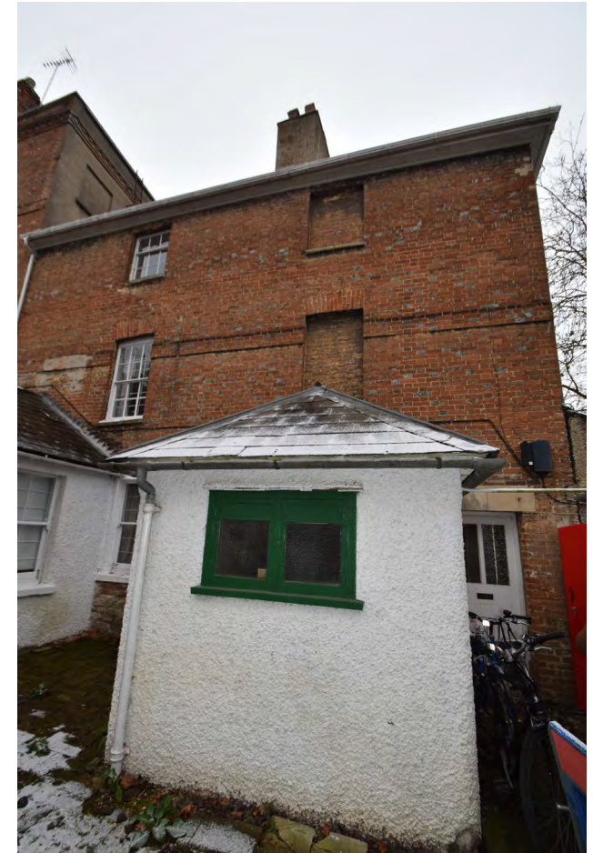
3.15 The north wall of the larder
