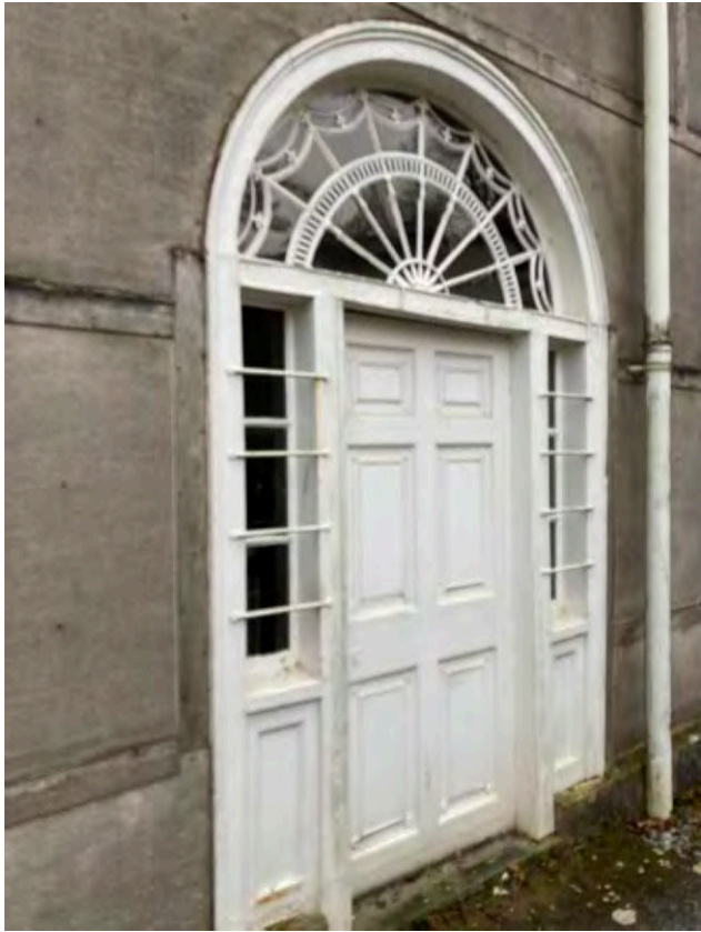
3.4 The front entrance
