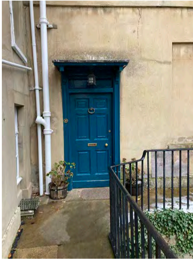
3.5 The entrance door at the rear of the main house
