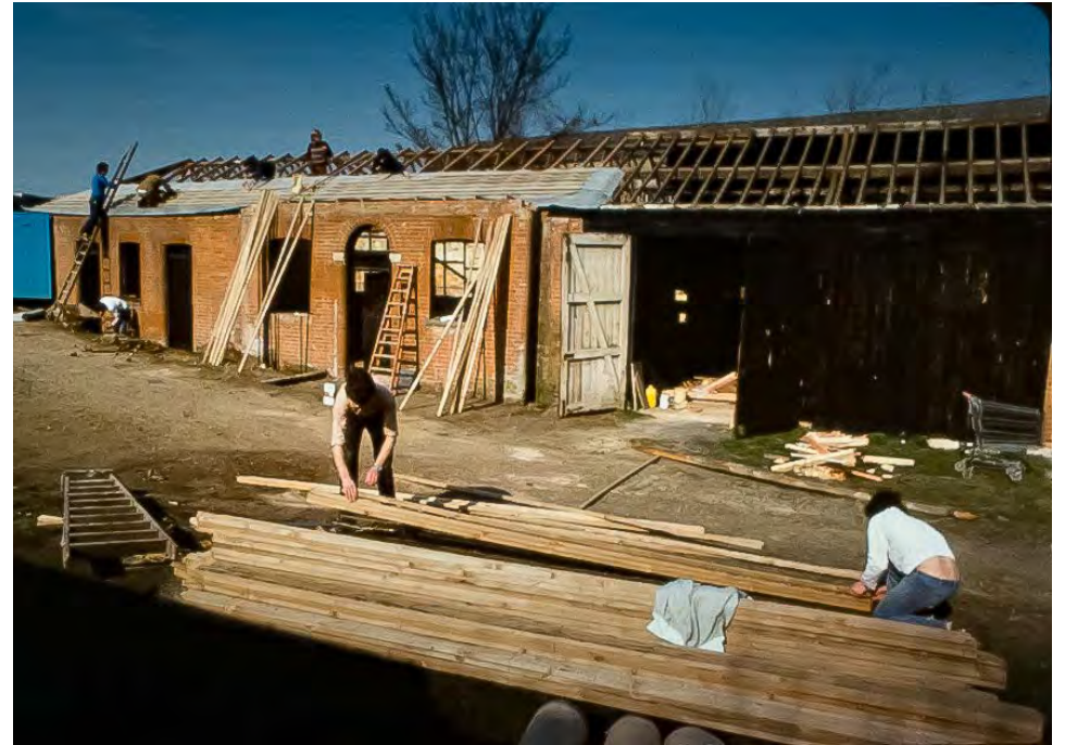
2.24 Replacement of the stable and coach house roof, c.1976 (Grandpont House archives)
