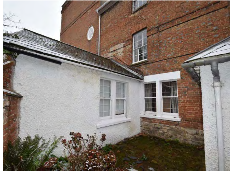
3.14 The west facade of the servants lounge (left)
