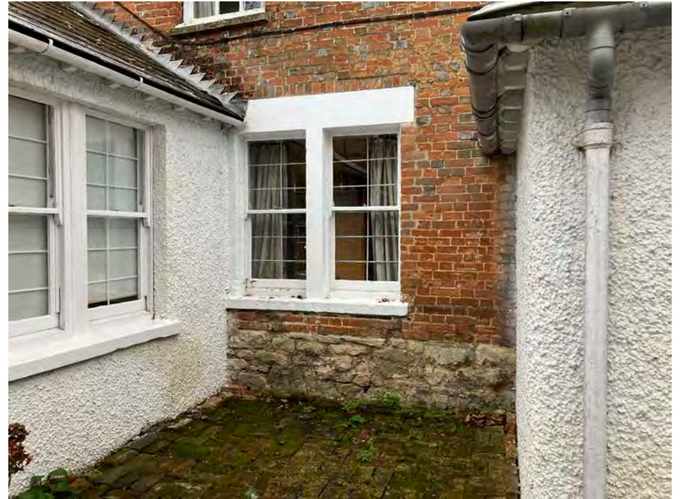
3.12 The base of the north wall of the west wing
