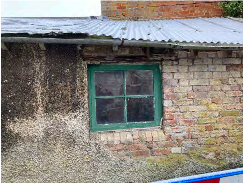
3.19 The east wall of the coal and wood store
