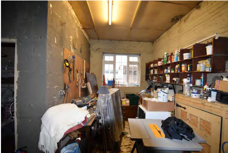
3.44 The coach house interior - A4
