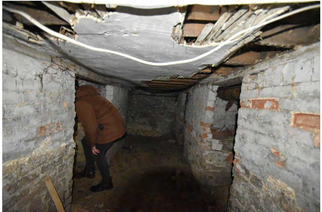
3.21 The basement at the north end of the house, looking east
