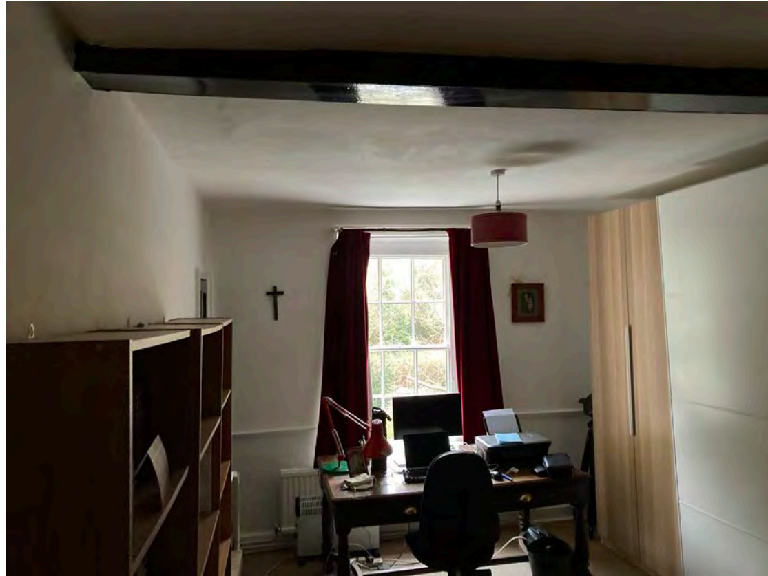
3.36 Room F9. The cupboard is on the left of the window
