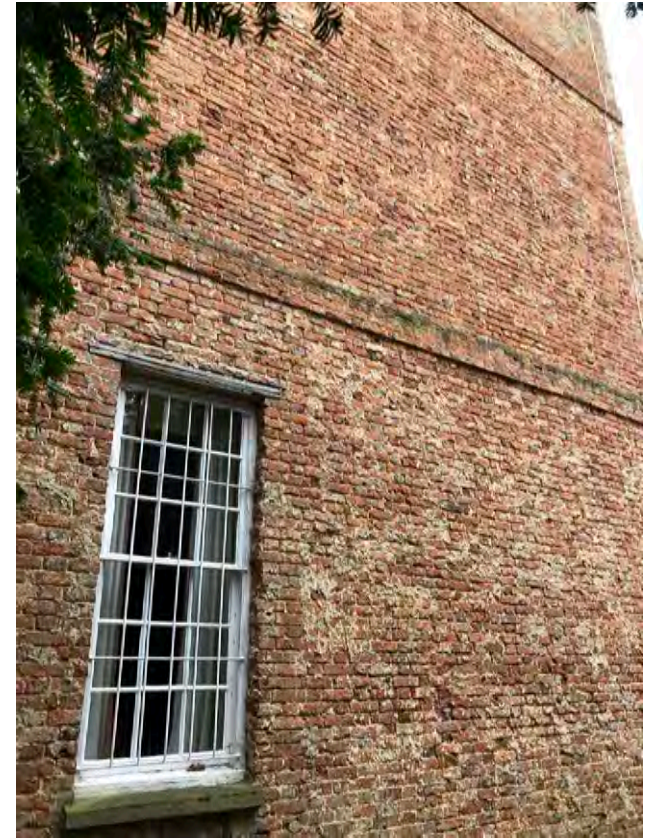
3.6 The south wall of the main house
