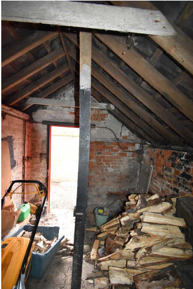
3.41 The coal and wood store - A1
