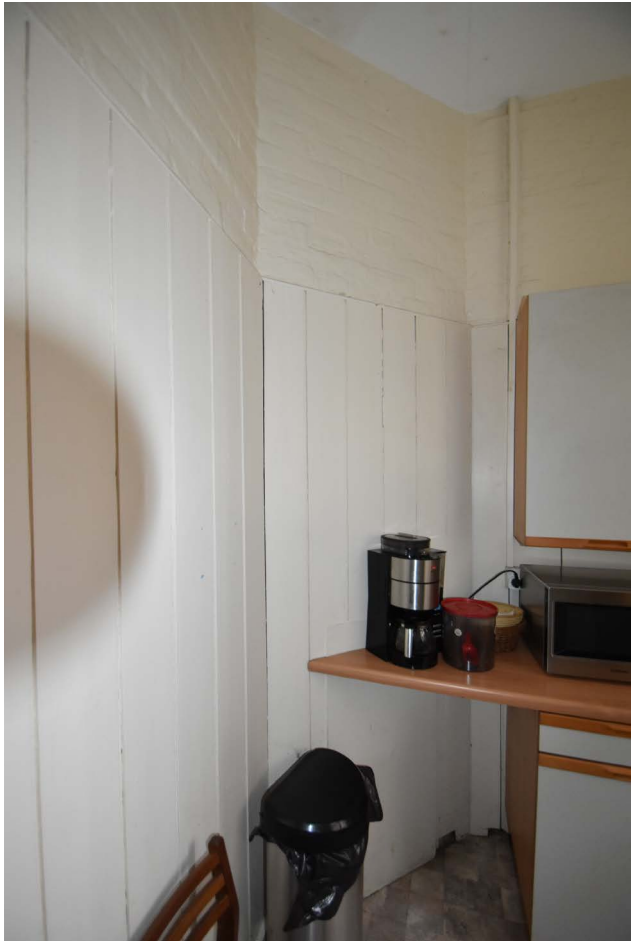
3.46 The kitchen with its boarded walls
