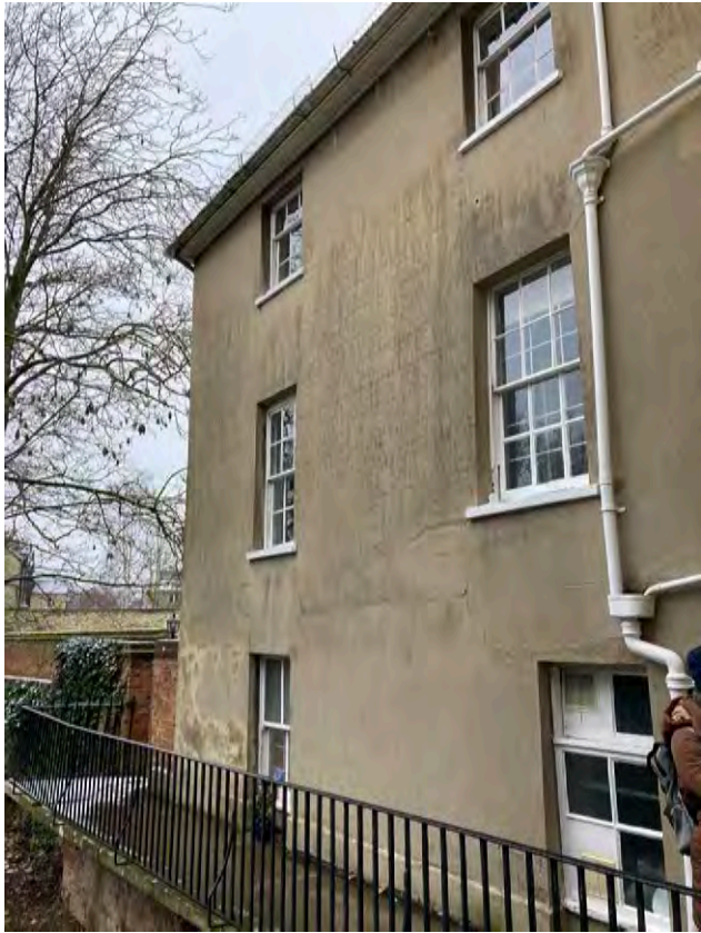
3.9 South wall of west wing
