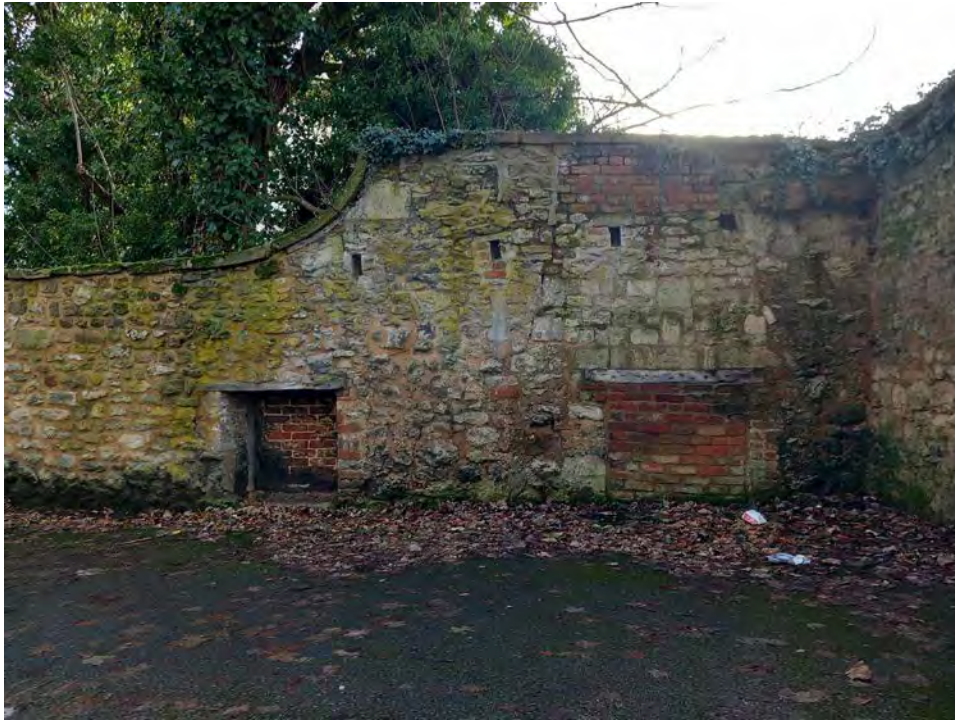
3.49 The internal south wall of the now demolished lodge
