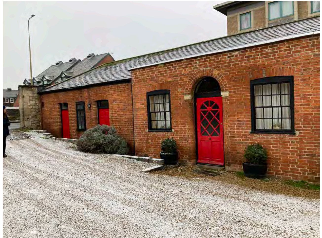
3.16 The south facade of the outbuildings - Stables (left) and coach house (right)
