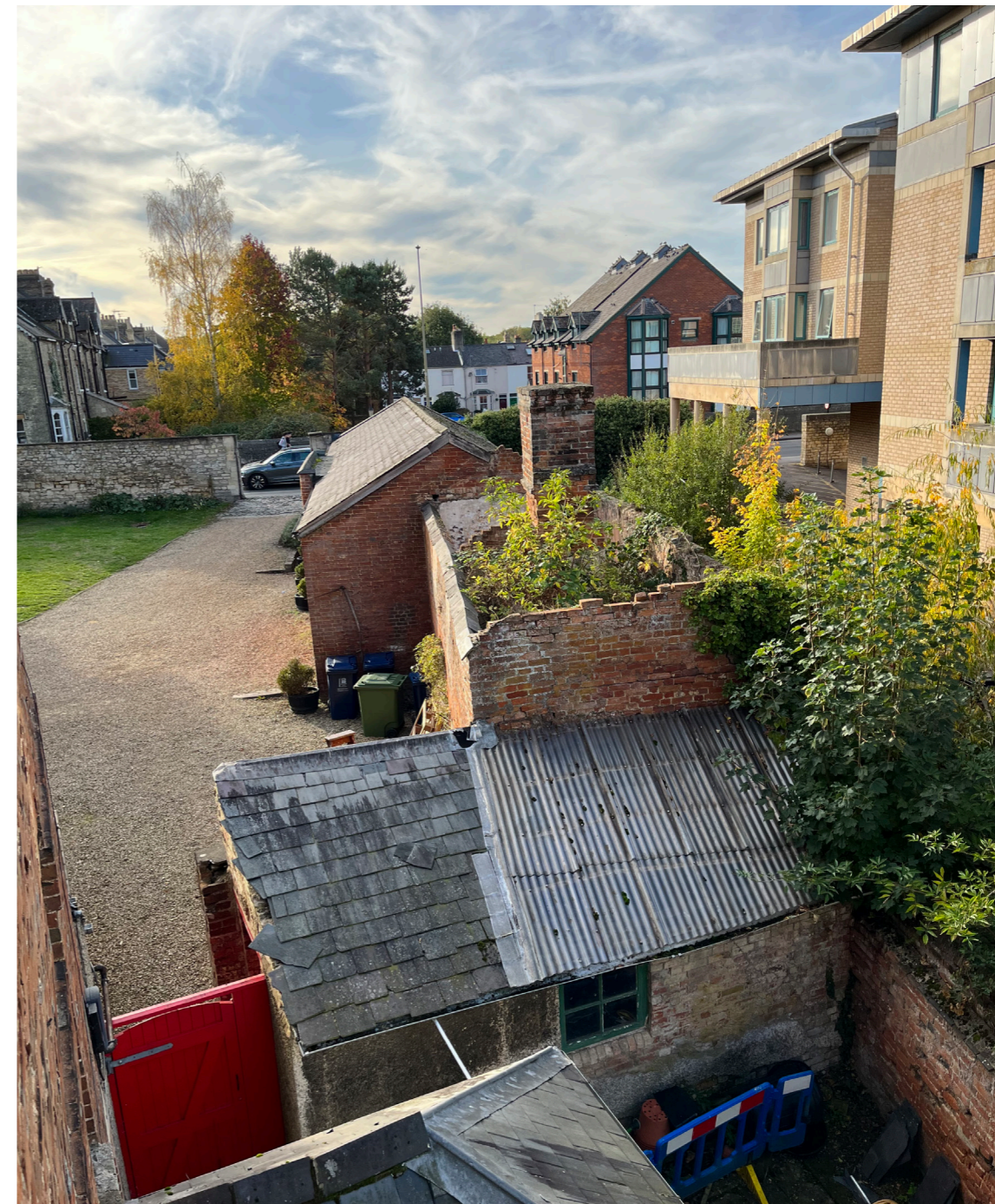
Image 21: External view facing west of north service yard, ruined servants cottage, stables block and entrance yard
