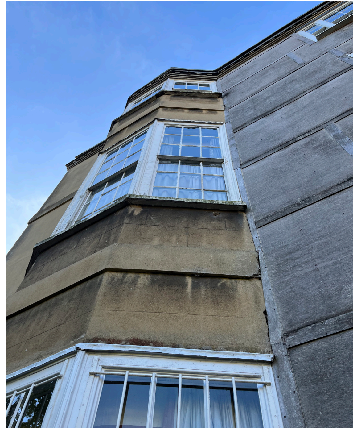
Image 23: External view of east facade canted bay with surviving render and adjacent plywood paneling
