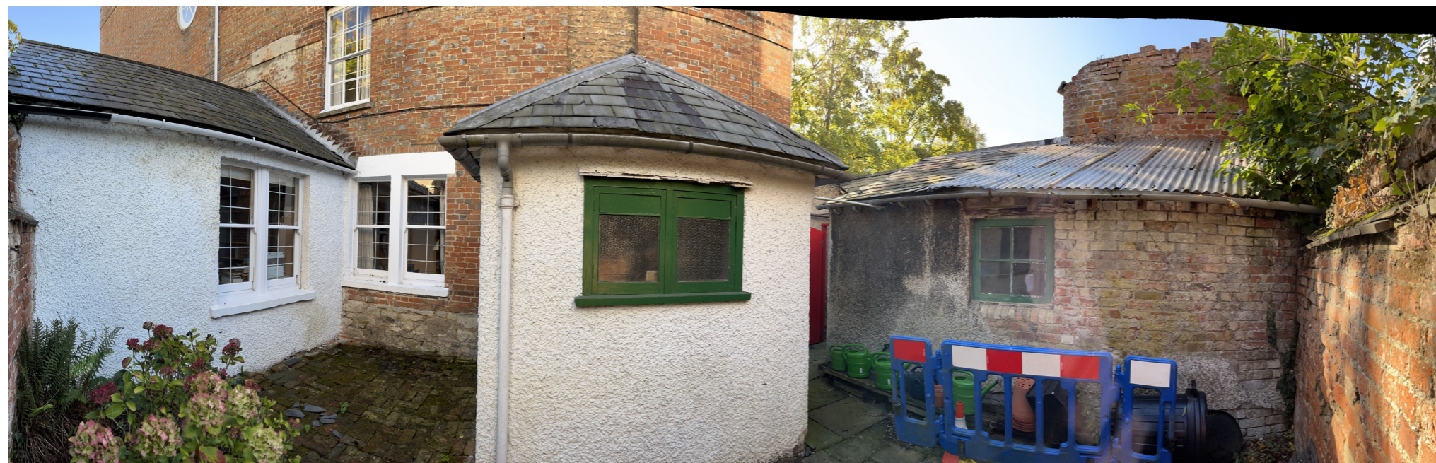
Image 19: View of north service yard 20th c. additions
