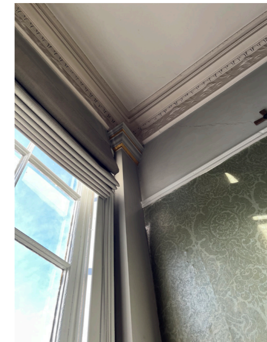
Image 14: Detail view of later addition decorative pilaster
