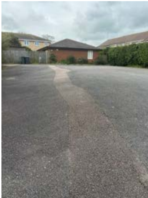
Photo 7: View of car park to caretaker's (showing repair to tarmac)
