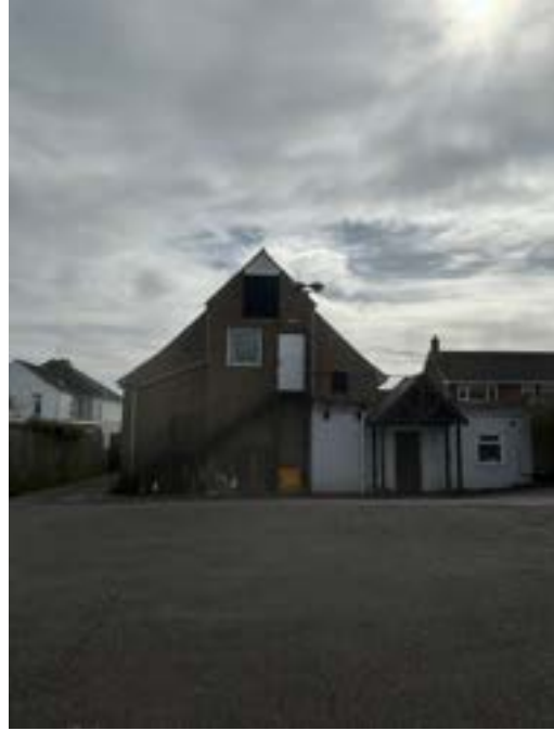
Photo 6: Rear of building from car park
