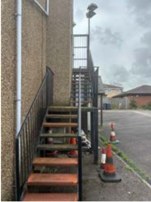
Photo 5: Metal staircase–rear of building
