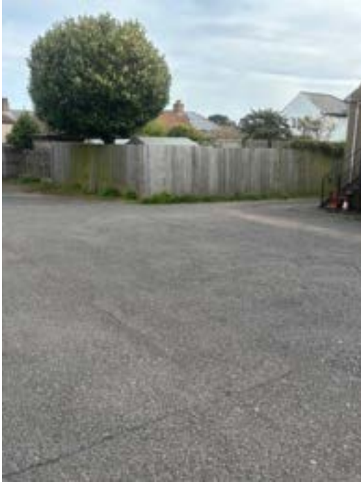
Photo 9: Car park showing tarmac ‘joints’
