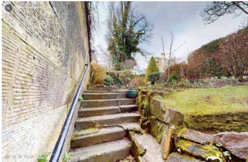
Existing Garden - North side of wall
