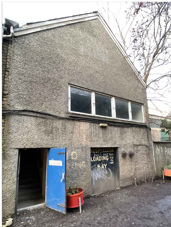
R001 - Rear Access to Basement
