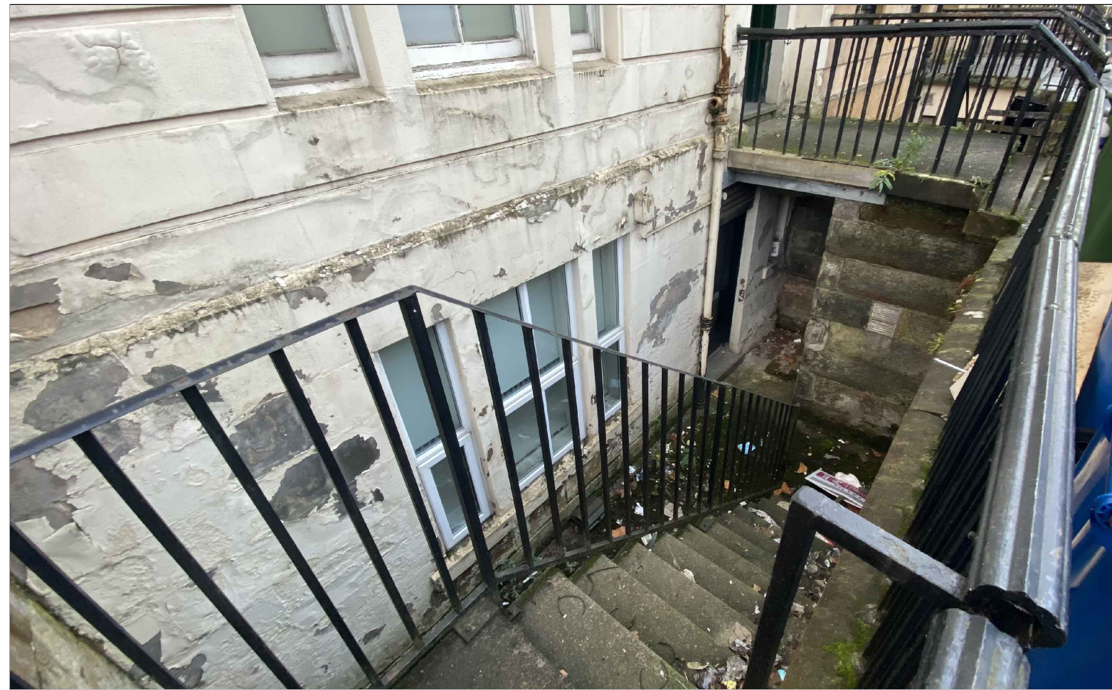
F002 - Front Lightwell and Basement Level Entrance
