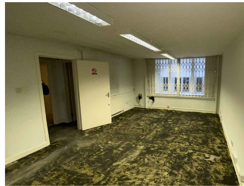
B005 - Front Office Space
