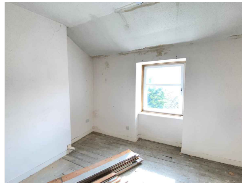
S003 - Second Floor Rear Office
