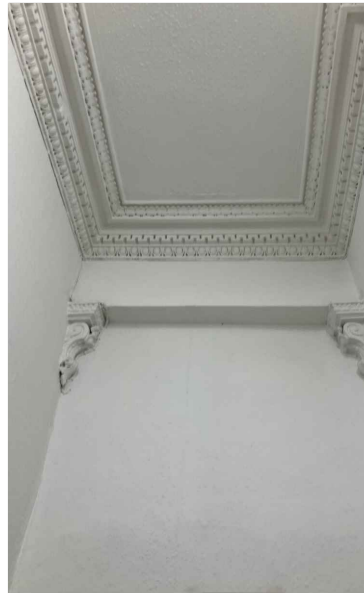
G003- Cornice to Entrance Hall
