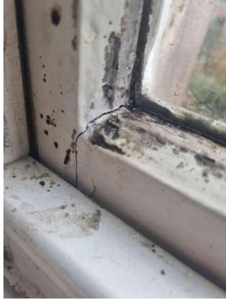
Internal woodwork is deteriorating and soft to touch. The second photo is of the tenon joint which is splitting.
