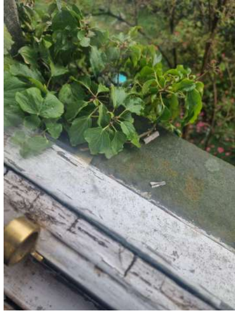
Seals and putty are failing to the windows.
