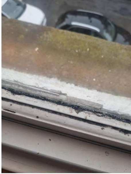
Failing external putty and deteriorated seals
