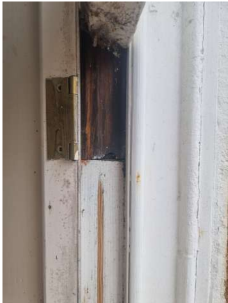
Rotting casement woodwork and midrail
