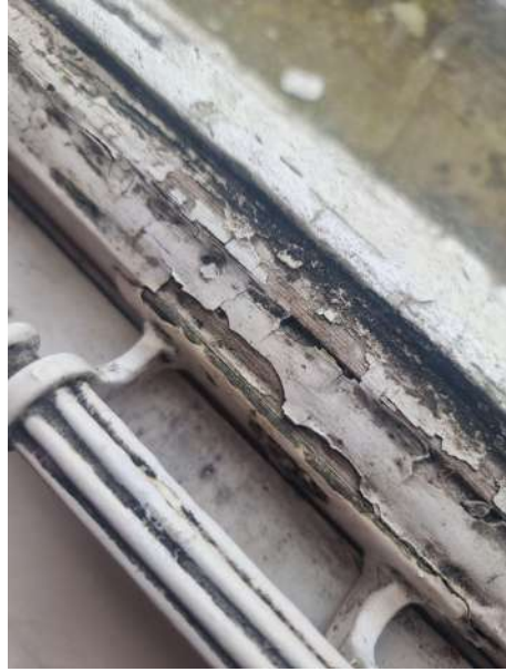
Failing external putty and deteriorated seals
