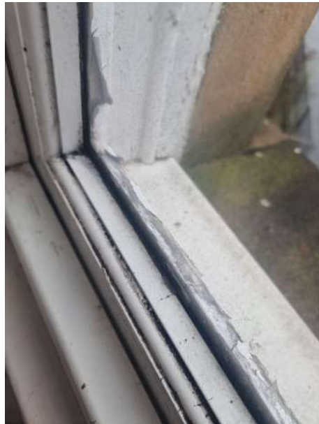
Rotting casement and external putty
