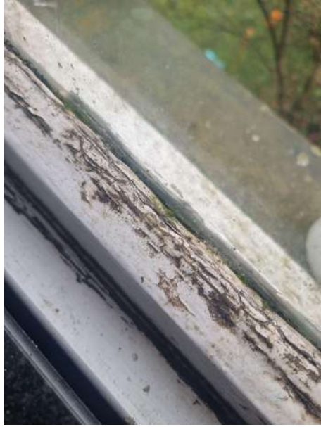
Seals and putty are failing to the windows.
