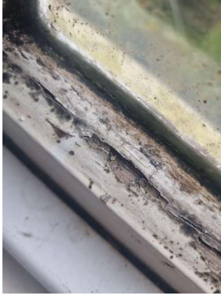
Internal woodwork is deteriorating and soft to touch. The second photo is of the tenon joint which is splitting.
