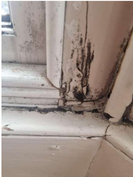
Rotting casement and external putty
