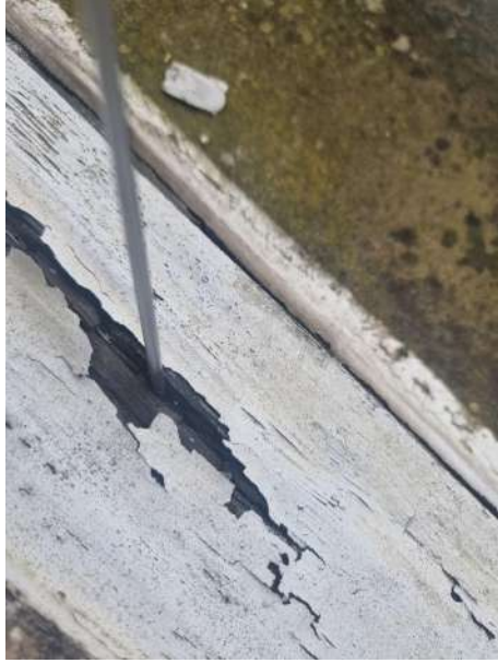
Rotten sill and failing tenon joint.
