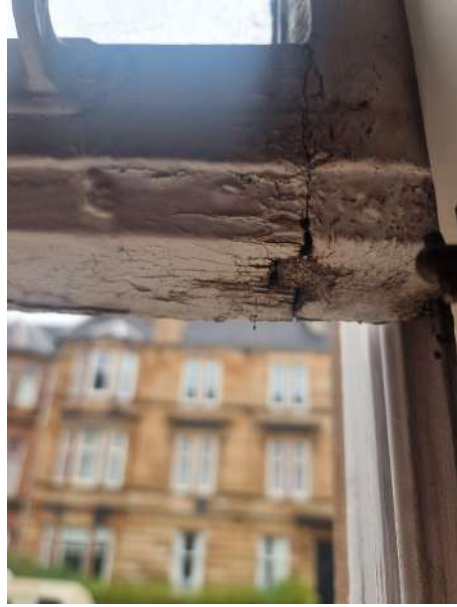
Rotten sill and failing tenon joint.
