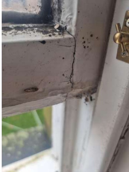
Splitting tenon joint.
