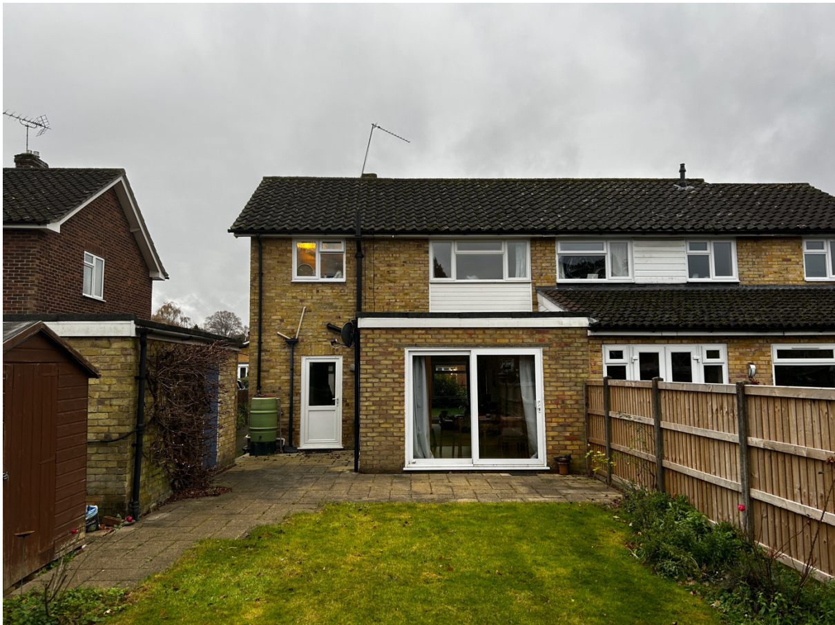
Rear of 17 Alton Road As Existing
