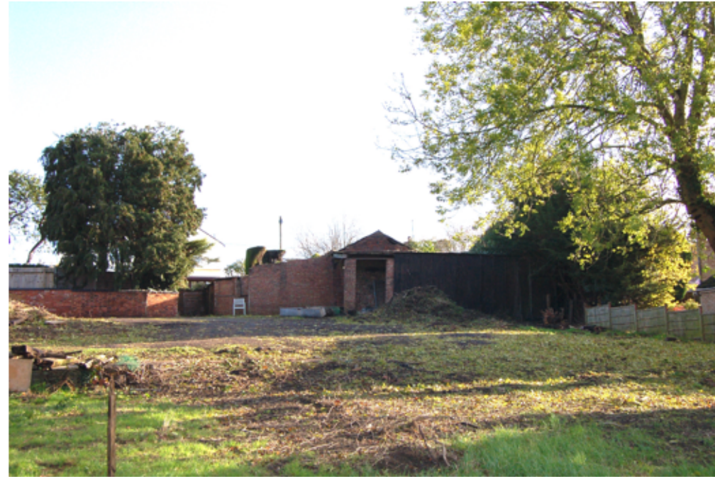
PS-002 B View from within the site looking east with the outbuildings surrounding the Smithy in the distance.
