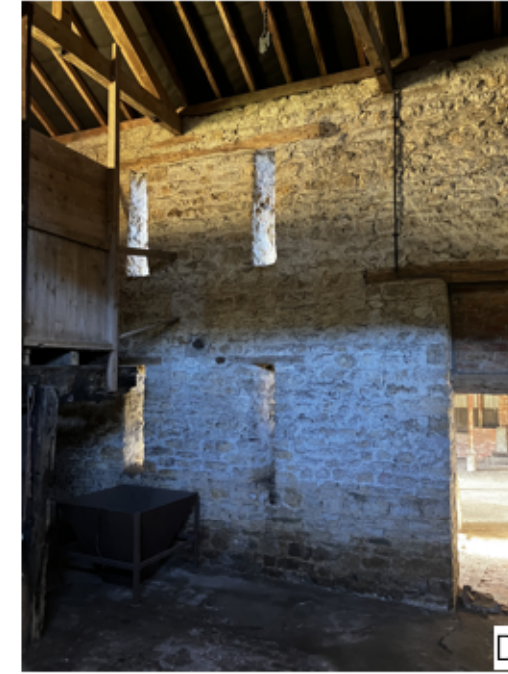
Openings on the west facing elevation.
