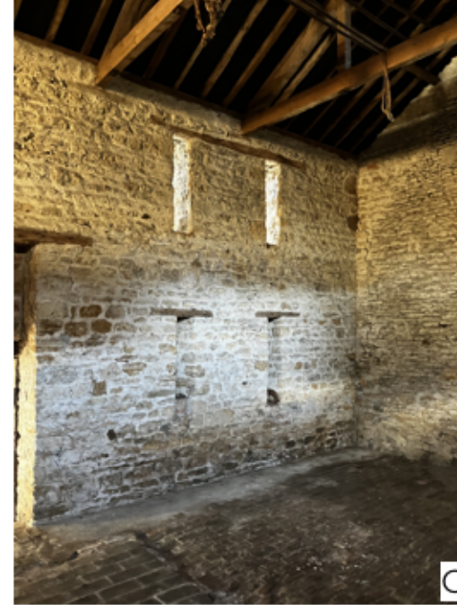
Openings on the west facing elevation.
